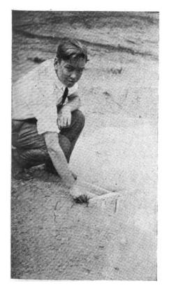
Fig. 8. Helper making sight on pavement. This sight is secured from the transit and permits lining up of transit without using helper again
