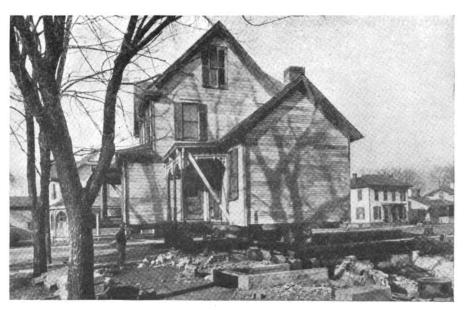
Fig. 3. Cribbing in Cellar for Trucks to Run On
