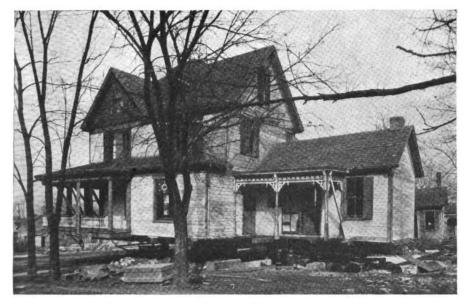
Fig. 2. Shows House Just Coming Out of Cellar for Removal
