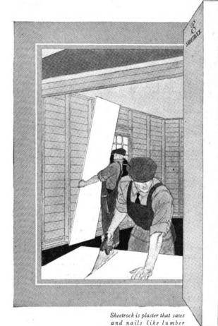
The actual thickness of a sheet of Sheetrock is 3/8-inch of pure gypsum plaster
