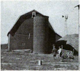
Figs. 5 & 6. This partial failure resulted from inadequate bracing after removal of cross ties for the purpose of opening up mow space.
