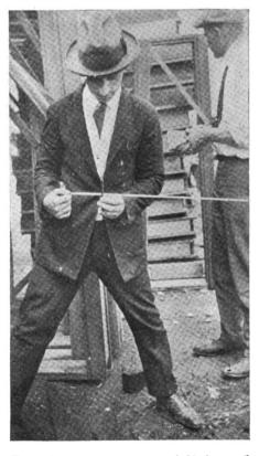
Fig. 3 shows the proper way to hold the pencil on tape in taking offsets from side of building. The zero end of the tape is held by the helper, while the rod-man holds and moves the pencil as directed by the transit-man.
