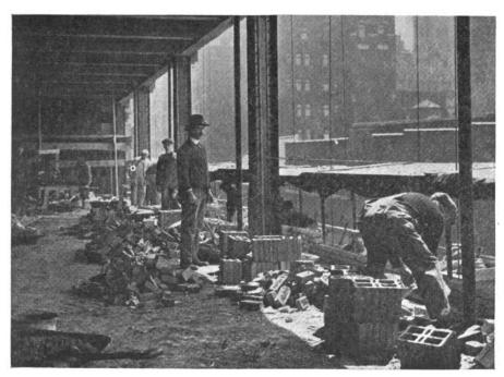
Improved Working Conditions on a New York Skyscraper. Safety and Comfort of the Bricklayers Have Been Attended to. Hanging Scaffold with Guard Rail and Overhead Covering Allow Men to Work with Maximum Efficiency—They Watch Their Work, Not Their Step. This Creditable Job is on the New York Times Building, Now Being Erected by the George A. Fuller Co., Builders, New York.
