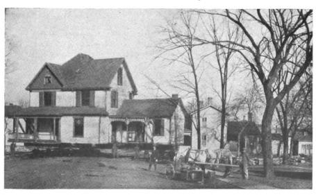
Fig. 4. House Out in Middle of Street Ready for Removal to New Site
