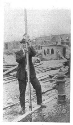
Fig. 3 shows the proper way to hold the level rod when taking levels. Figures are held toward levelling instrument so as to be easily read.
