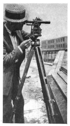
Fig. 5 Shows Method of Getting the Sight. Note Method of Focusing by Use of Screw on Telescope.
