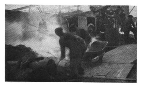
Concrete mixing in winter time is shown in this picture. Here the aggregate is being heated by being placed on metal pipe in which fire has been kindled.
