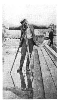
Fig. 7. Signaling the Assistant Line Is O. K. Note Position of Plumb Bob Over Cross Under Transit.
