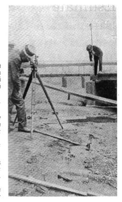
Fig. 1 illustrates the correct method of holding level rod on corner of uncompleted building to obtain first floor levels. Note level set up for taking readings.
