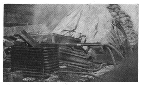
Hot water is necessary for winter concreting. Here it is being heated in pipe coils in which a fire has been kindled.
