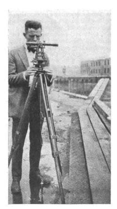
Fig. 4 Shows Correct Method of Leveling Transit. Transitman Manipulates the Thumb Screws,
