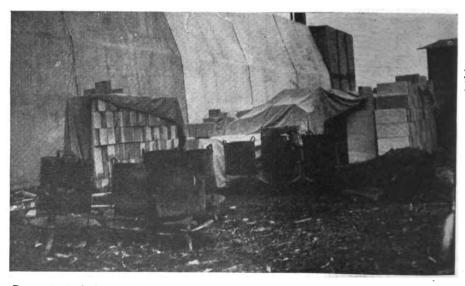
Preparation is the keynote of successful concrete work in cold weather. Here coke stoves are being put in readiness for heating enclosure where concrete block walls are being laid.
