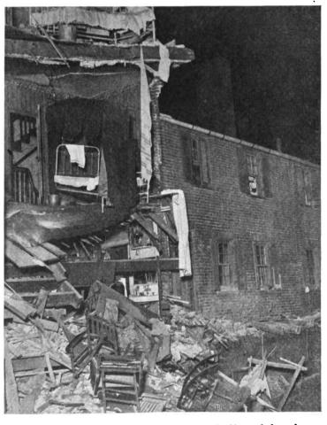
An example of property damage that contractors should guard themselves against by adequate insurance. Here a portion of the wall of the building adjoining the excavation for a new structure collapsed into the excavation. This particular accident occurred last September at Washington, D. C.
