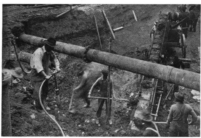
Compressed air picks can now be had that greatly reduce the labor of excavating in clayer soils. The laborers only need to move the materials to the automatic portable loaders which fill the carts rapidly. Machinery will cut your excavation costs.
