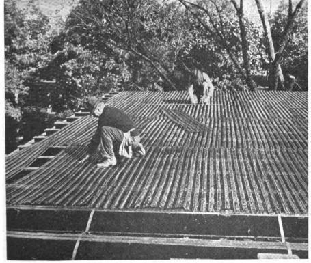
Method of Floor Construction-Metal Lath Being Attached to Steel Joists
