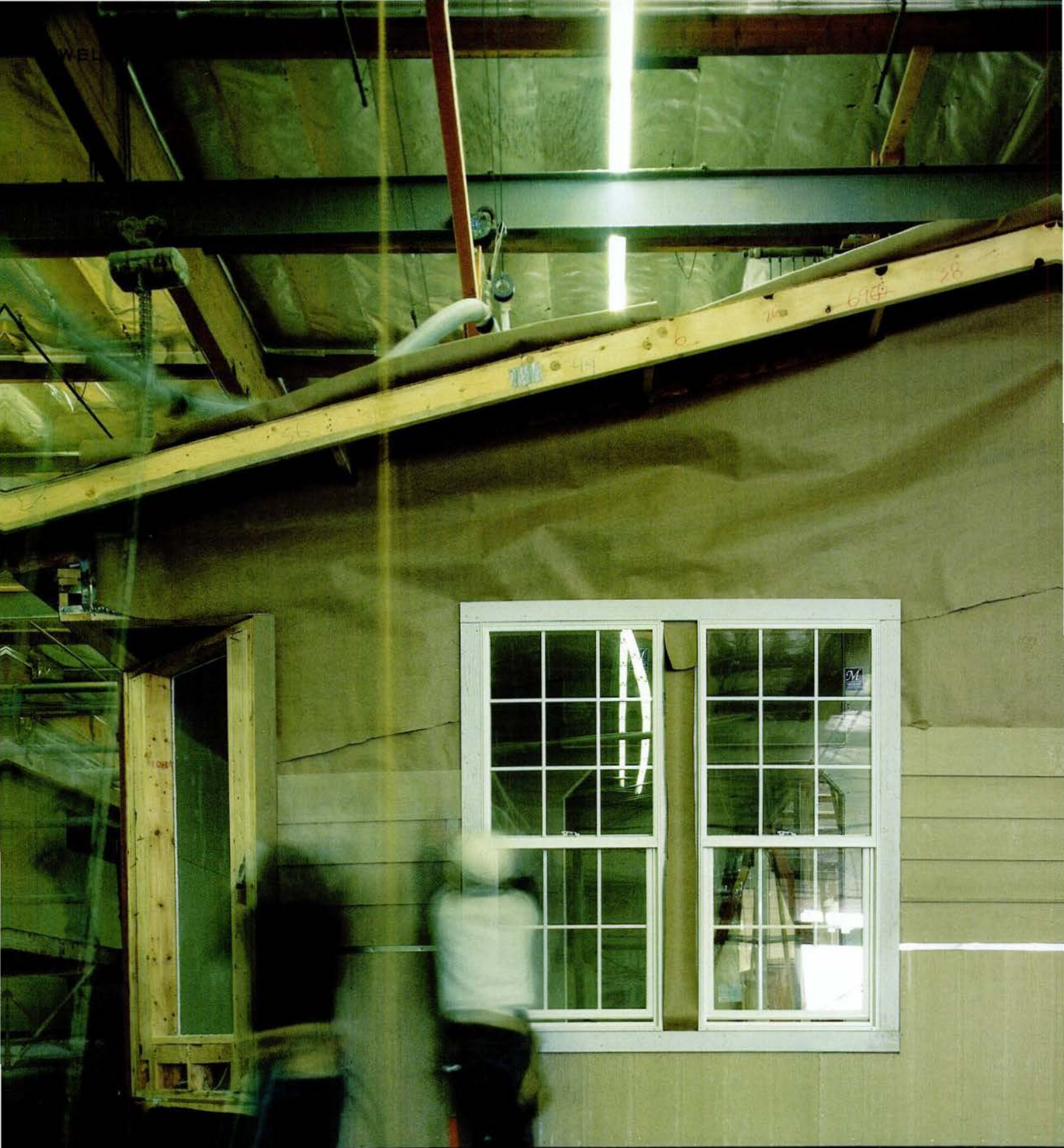
Woodland, CA: Silvercrest Western Homes manufactures three houses every day.
