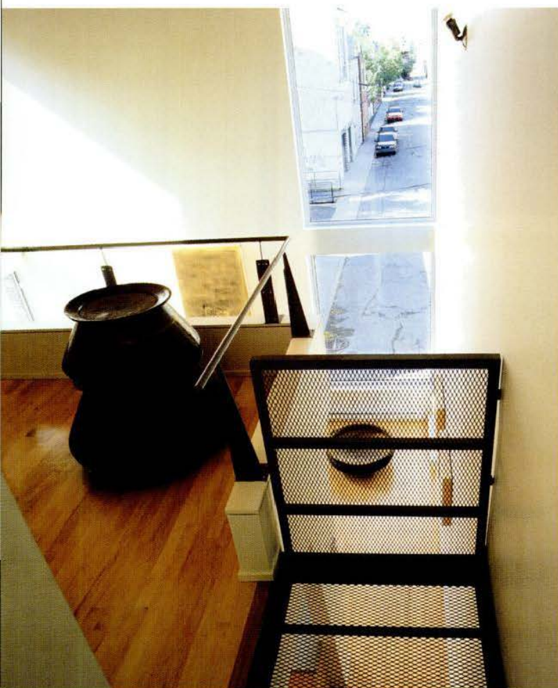
A 36-foot-high metal stairwell with industrial skylight connects the house's three levels—a ground-floor studio, vast living/dining/kitchen area, and a third-story bedroom with bath.
