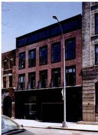
The landmarked two-story garage (top) in 1994 before Seggerman and company got their hands on it. Below, the façade as it appears today.
