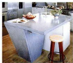
Kitchen counter and vertical panels. Trowel finish.
