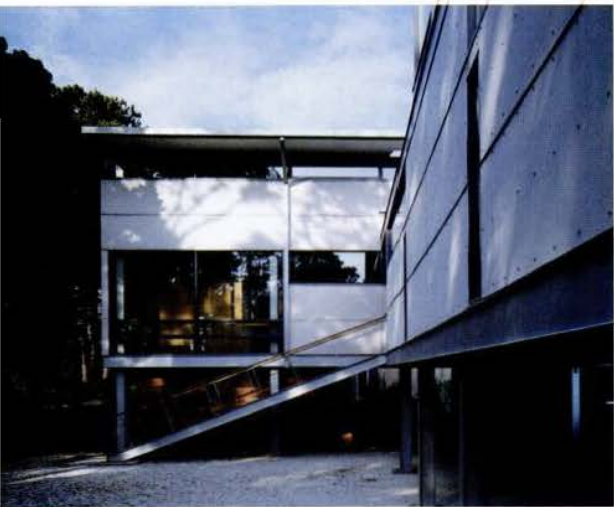
The Robinson house is entered through a main door on the second floor, which is reached by an exterior steel staircase with cedar handrail. Photo by Richard Leo Johnson. A notated plan of the first floor is shown at right.
