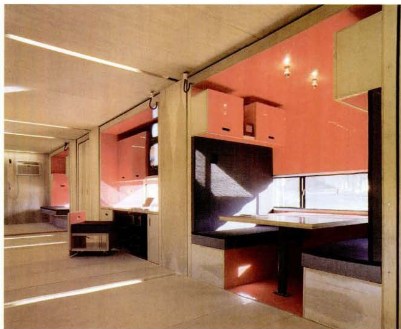
Right: The bedroom, study, and dining areas slide in and out of the shipping-container body for easy transport.
