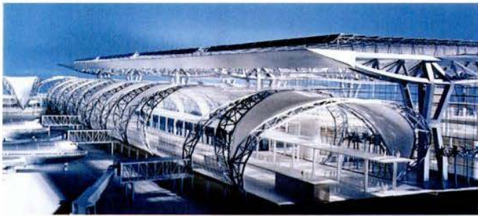
Models of Bangkok's new airport, scheduled to open this year, show the complexity of the roof, which ventilates the vast
