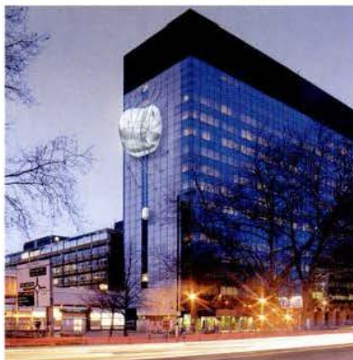
The Web House / By m3
