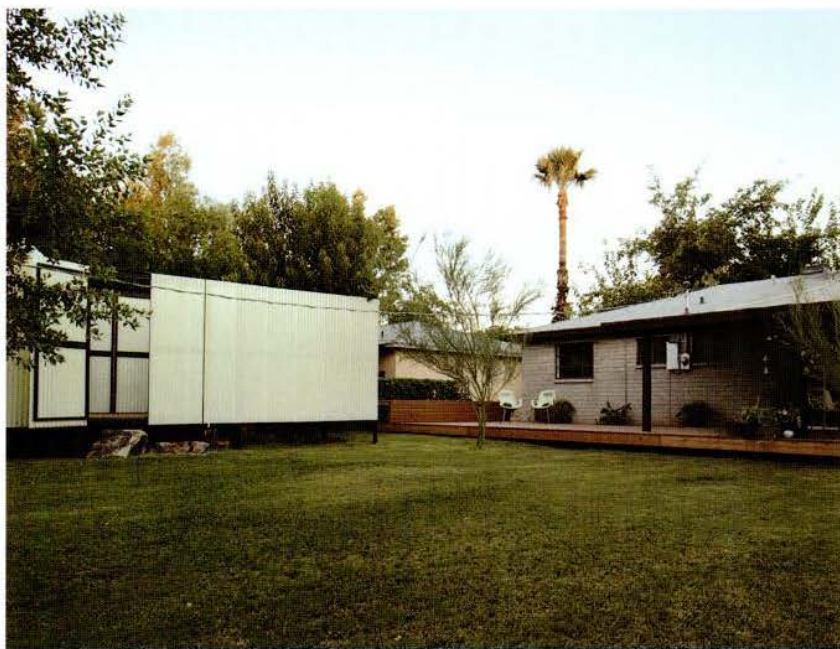
Portable and easy to move should the couple relocate, the pods rest lightly on the lawn behind the main house.
