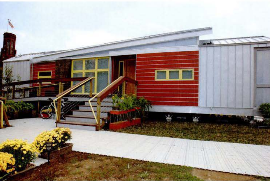
The University of Colorado's BioS(h)IP is named for the team's invention, a recycled wastepaper-and-soy insulation system called Bio-SIPs. After nine days of competition, it won first place.
