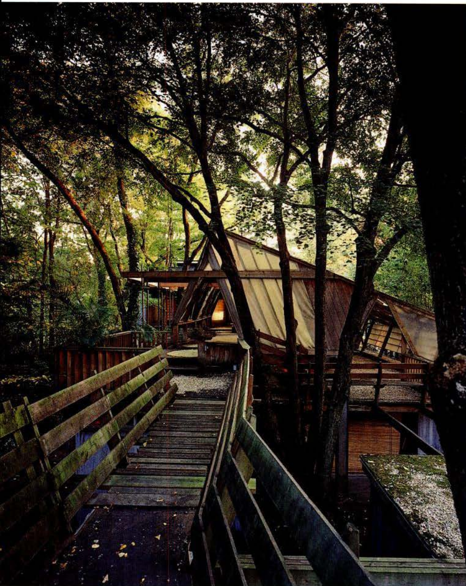
A catwalk (left) leads to the meditation zendo in the roof garden. The hand-hewn spiral staircase joining garden and deck (below left) provides structural support. Below right is Rose's mother's sitting area.
