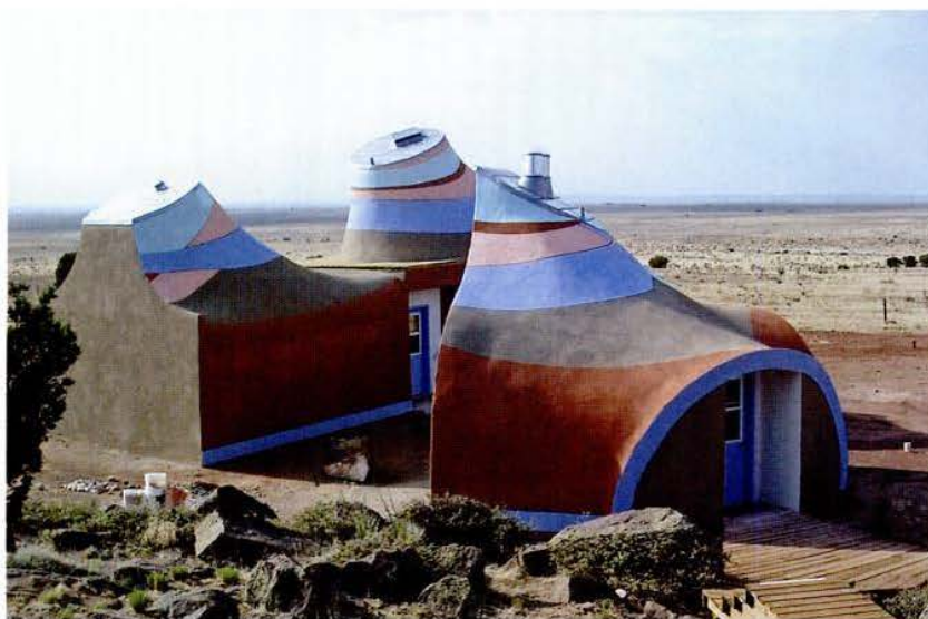
Kasuba's latest creations are a series of small, eccentrically shaped buildings in the desert of New Mexico. The first version of her studio and kitchen buildings (left) were painted with bands of color. The final version of the kitchen (right) is clad with aluminum shingles that reflect the desert sky.
