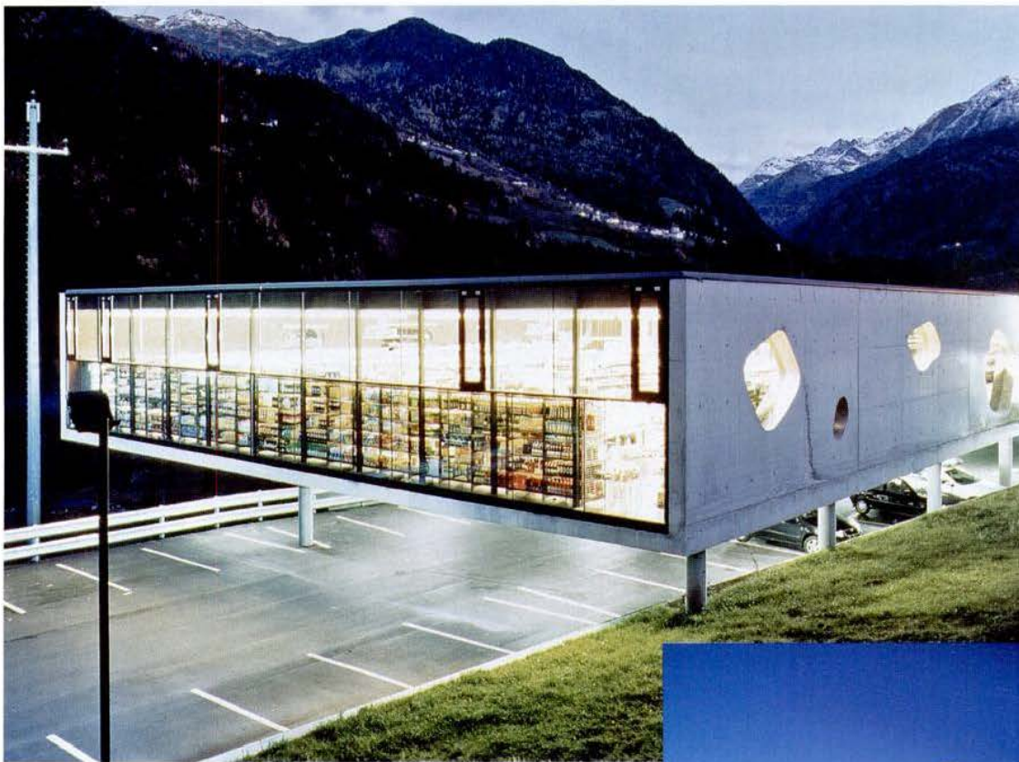
MPreis's outpost in Wens (top), tucked deftly among the Alps, was designed by Astrid Tschapeller and Rainer Köberl; the elevated concrete market is reminiscent of Le Corbusier's Villa Savoye. The store in Wattens (bottom left) opts for live trees over stripped trunks, and the glassy store in Fügen (below right) by Helmut Seelos positively glows at night.
