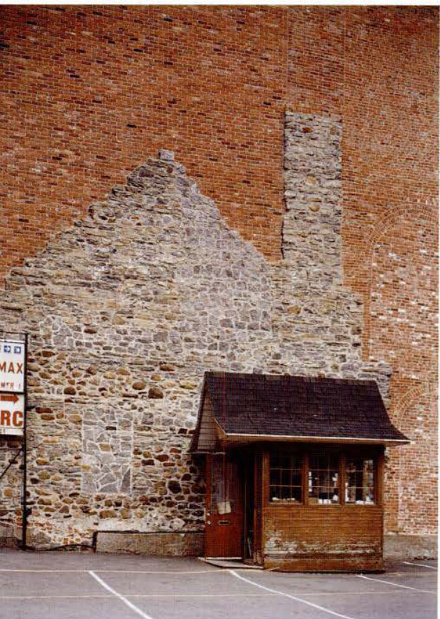
Matthew Monteith captured a small parking kiosk—a mere shadow of the former structure—on the Rue St.-François-Xavierut in Montreal.
