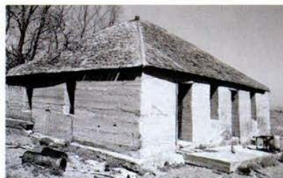
1903 Burke House, Nebraska The oldest-known extant straw bale home in the U.S.
