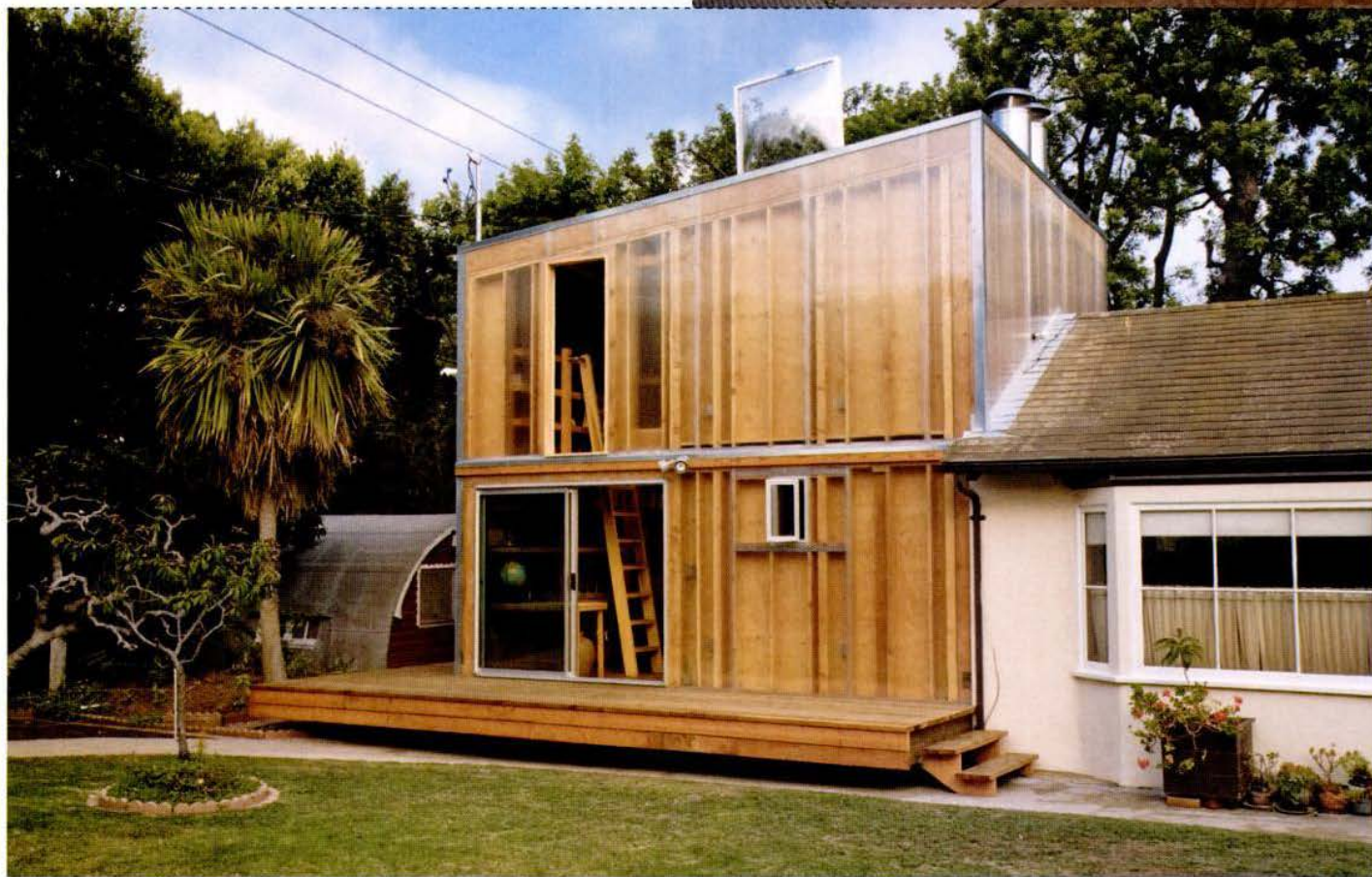
Photos by Joshua White (exterior), Michael Wells (interior)
