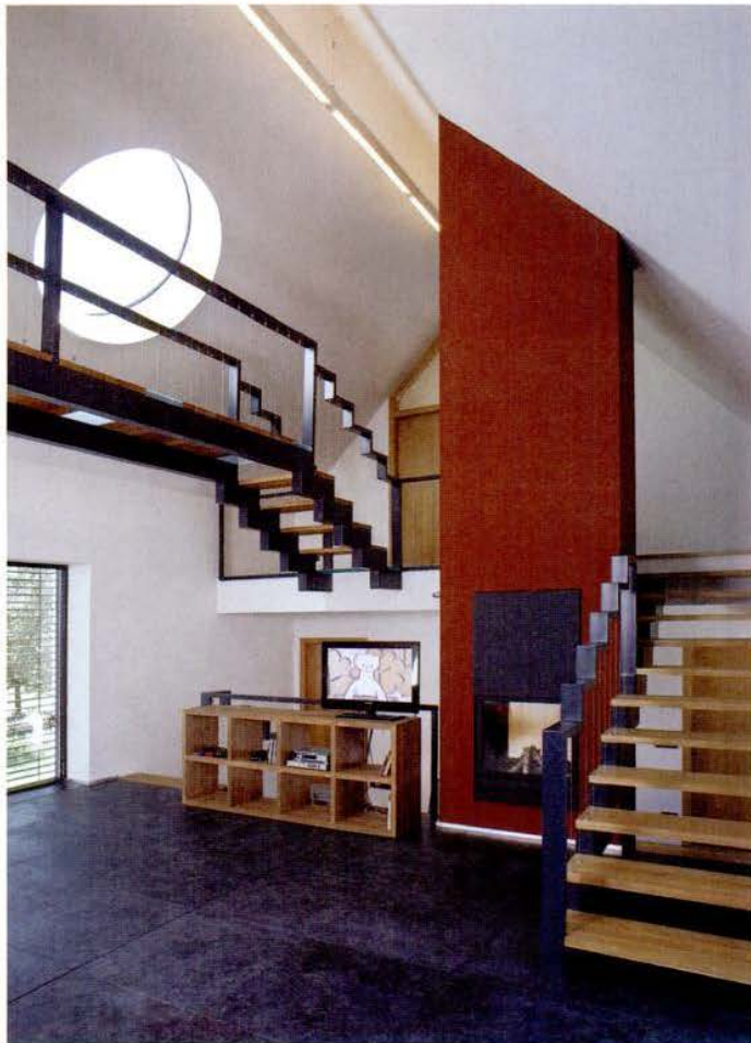
Circular “sun disks” cut into the slanted roof create light shafts that move throughout the day, casting angular shadows as they pass over the steel staircases and catwalk.
