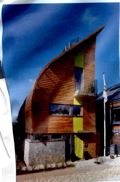
Curved roof of the Lighthouse in London in sunlight and catches the wind in to passively light and cool the house.
