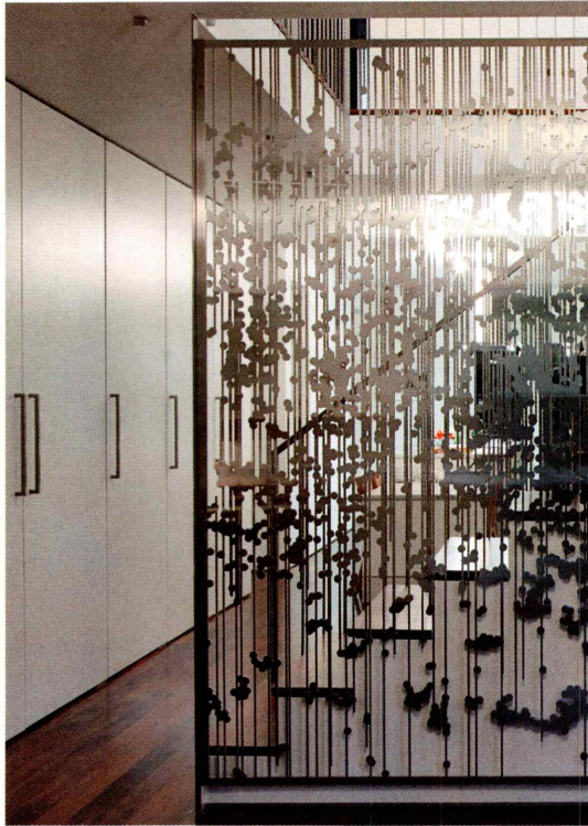
Andrew Magnes's hanging screen (this page), composed of aluminum circles and lines, cut with a CNC water jet, separates the entry from the staircase and rear kitchen area. To accommodate his passion for cooking, Renaldi (opposite bottom) insisted on the long Carrara marble countertop, a niche for cookware (opposite top left), and ultra-contemporary appliances.
