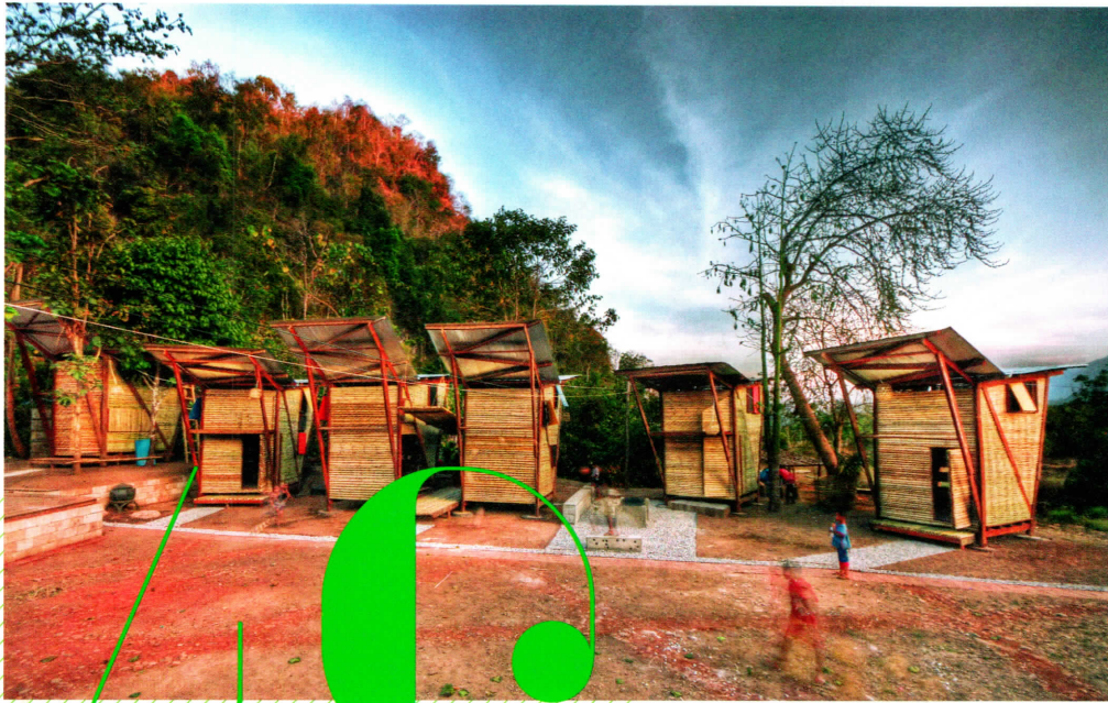
The Soe Ker Tie houses provide lodging for around 50 orphans on the Thailand-Burma border. They were constructed using local materials, including ironwood and woven bamboo. The roofs promote ventilation and collect rain.
