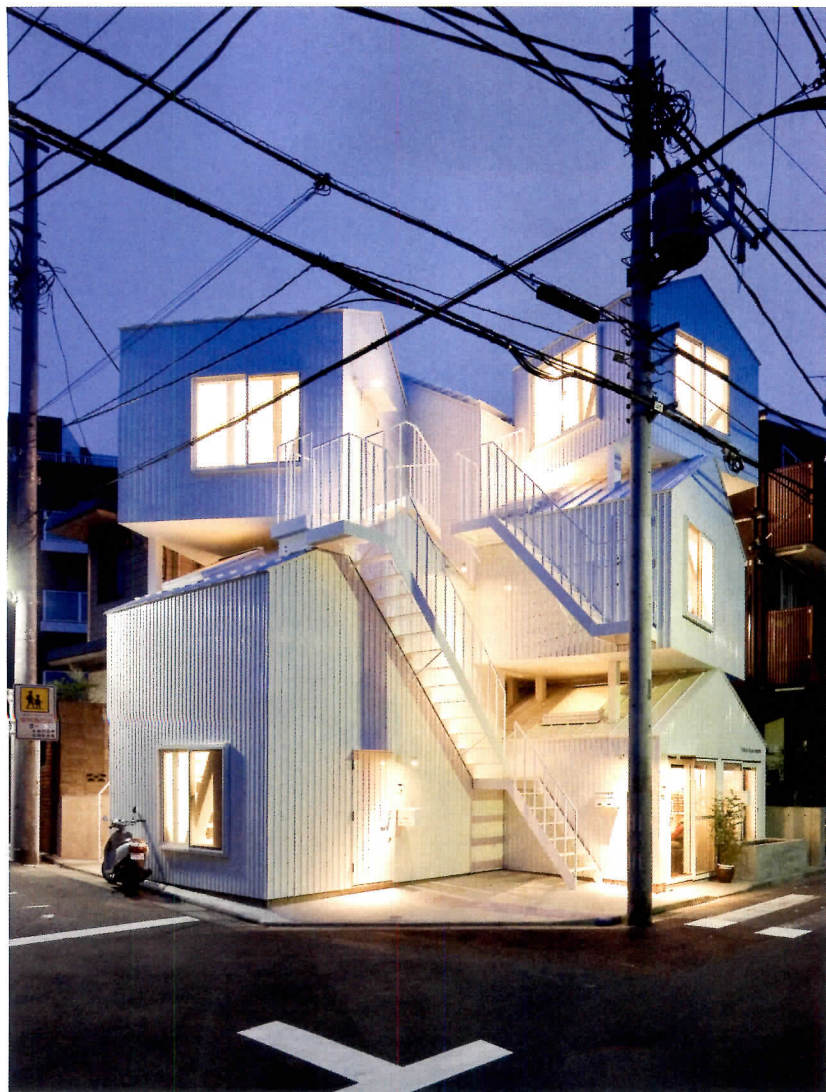
Resembling a jumble of houses piled on top of one another, the dynamic Tokyo Apartment building from 2010 (above) evokes the chaos and crowding of Tokyo. Adding to the complexity, the dwelling units do not correspond to the house forms. Instead, stairs and ladders link individual tenant spaces that span the different pitched-roof volumes. The building sits on a corner site amid a quiet residential neighborhood. In 2008, Fujimoto designed House N (left), one of his first commissions, for his in-laws.
