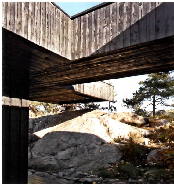
◀ A section of the roof reaches over a rock outcropping—a detail that visually connects the house to the landscape and offers a handy way to climb up to the roof deck without using a ladder. ■■■
