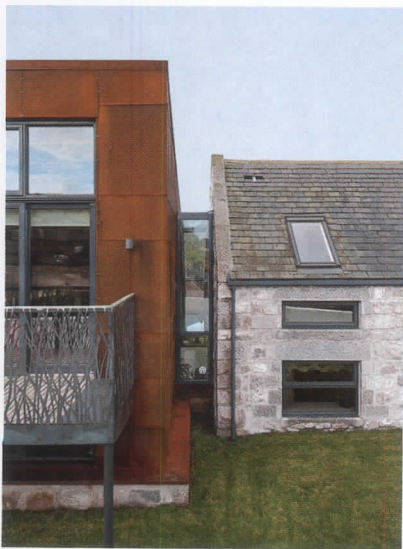
Cor-Ten steel from a ship building yard clads the new structure, which connects via a glass “bridge” to a rebuilt stone farmhouse containing the bedrooms (above).
