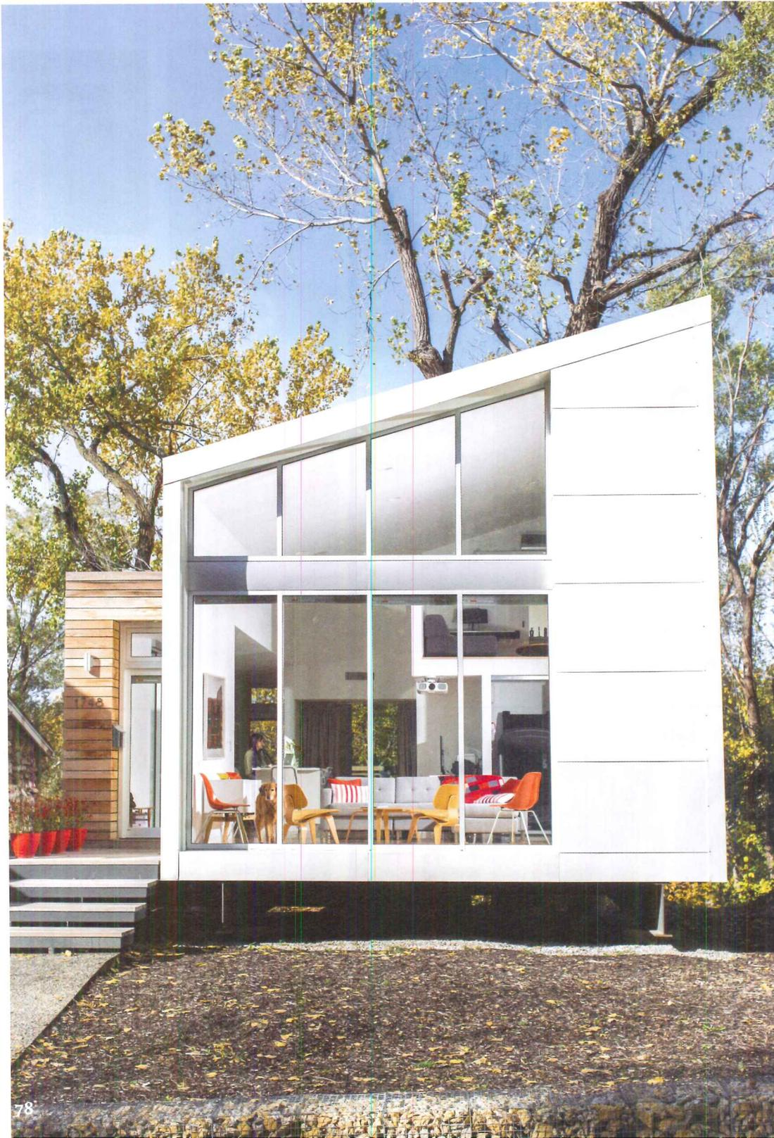
The house that Kem Studio designed for Sarah Magill on a narrow lot in Kansas City has a steel facade with reclaimed cypress cladding near the entrance. The entire structure sits atop a steel foundation set on concrete piers that were driven into solid stone.
