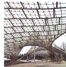
Olympiapark, in Munich, site of the 1972 Summer Olympics, still hangs together thanks to the tensile canopy designed by Frei Otto and Günter Behnisch. Munich, Germany 1,803 likes
