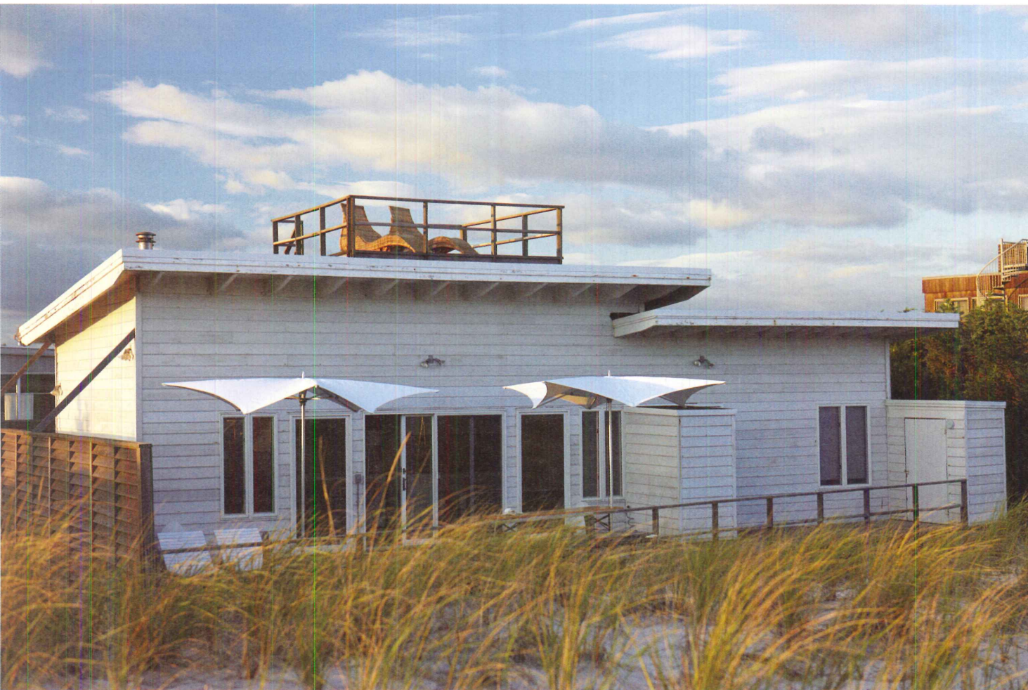
The wood screen concealing the outdoor shower (above) was painted yellow and white, matching the color scheme in the guest bathroom. The steps lead to a roof deck (below), where the owners can enjoy sweeping views of the ocean.
