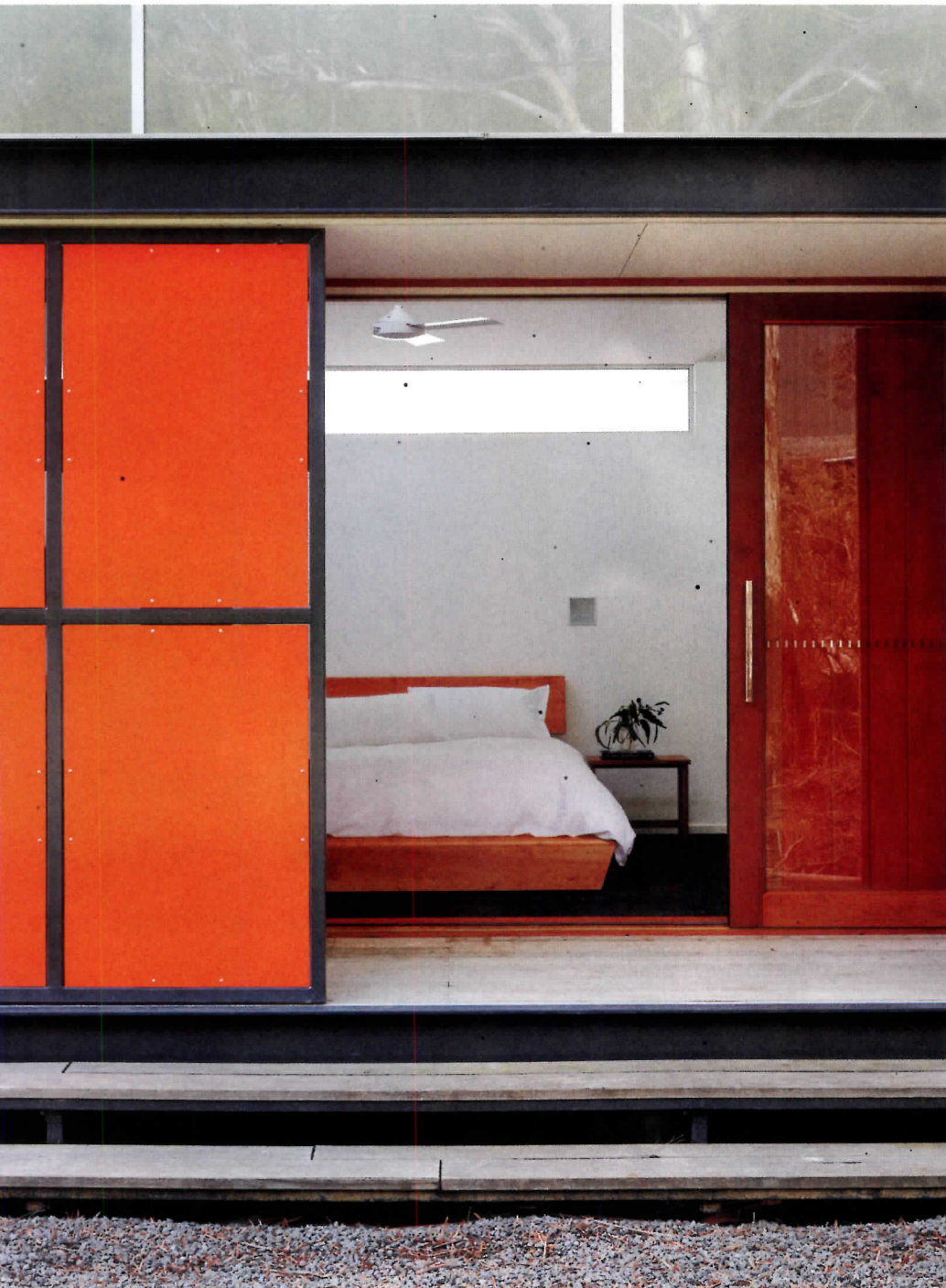
The home's double-skin structure makes the most of Tasmania's variable climate. Both sets of panels slide open for maximum views and solar gain; in inclement weather, they shutter completely, while clerestory windows bathe the space in light.
