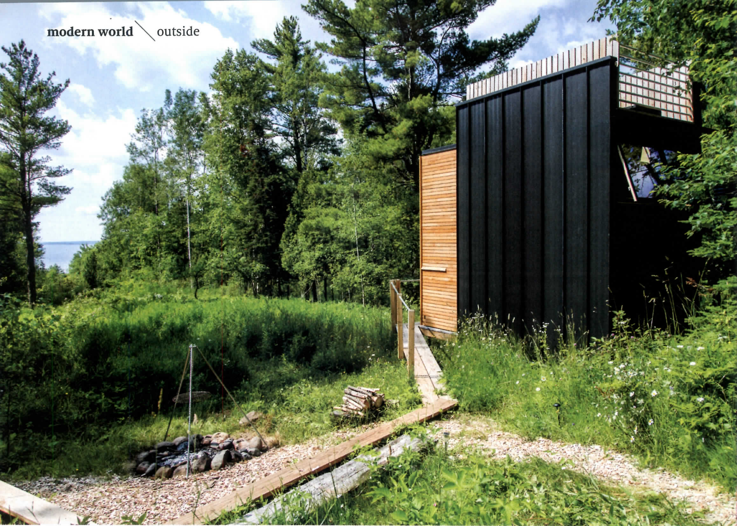
A standing-seam steel roofing panel clads a portion of the exterior (above), while the aluminum pipes also serve as the railing for the roof deck. The family cooks all their meals at the fire pit outside.
