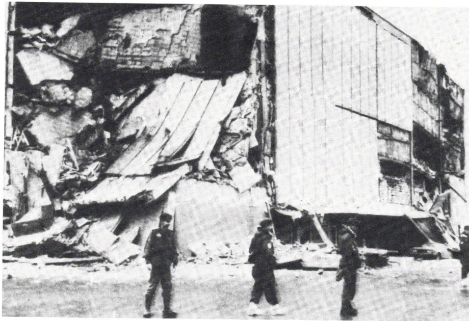
MASSIVE CURTAIN WALLS FELL OFF THIS ANCHORAGE DEPARTMENT STORE FAÇADE
