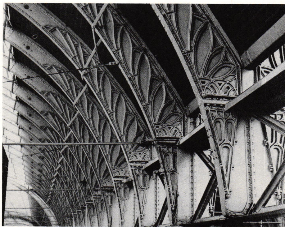
RIBS SUPPORTING ONE OF THE NAVES AT PADDINGTON STATION, 1852–1854.
