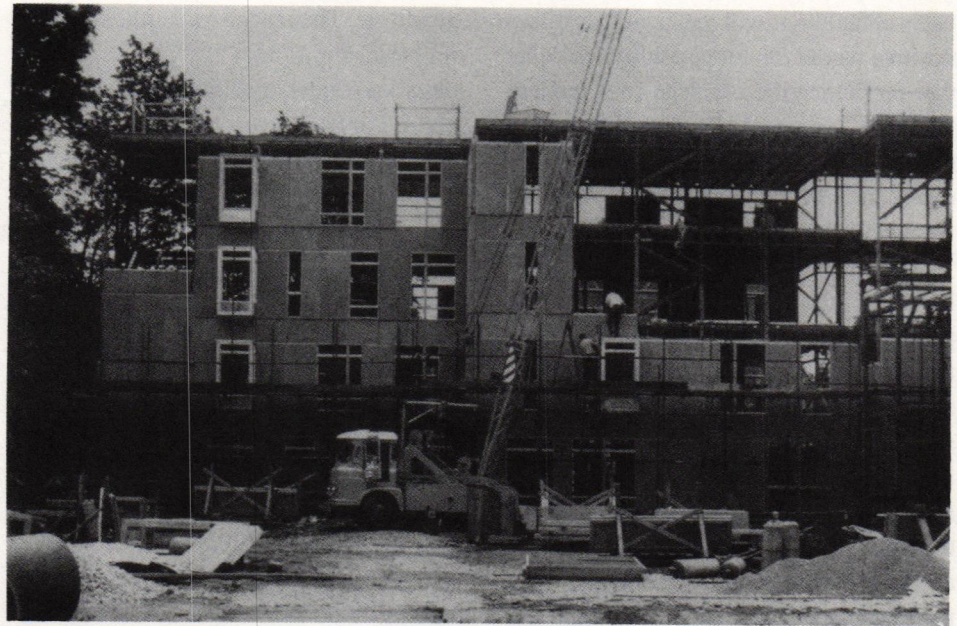
Wing of Derwent College under construction. With the roof deck on at an early stage, the contractors can proceed with cladding and other tasks unimpeded by bad weather. (From Toward a Social Architecture ; photo by Sir Andrew Derbyshire.)
