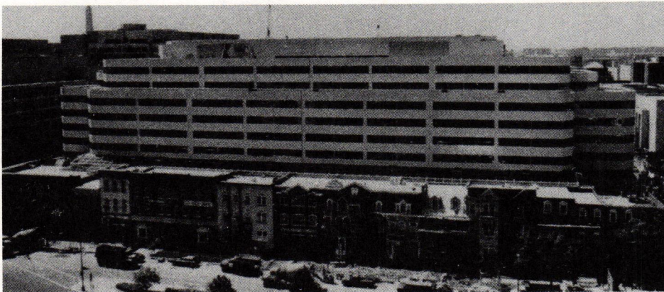
A façade preservation project in Washington, D.C.: the front section of a row of townhouses was preserved and separated from the new high-rise office structure to the rear by an atrium. (From American Mosaic ; courtesy George Washington University.)
