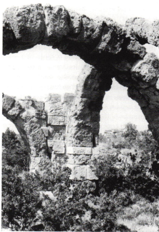
Bath-gymnasium at Alexandria Troas (modern Turkey), which dates to the middle of the 2nd century. Restored plan by Fikret Yegül (after Kolderwey and Smith), and present-day view of the ashlar arches connecting the corner piers of the square central hall, labeled P on the drawing. (From Baths and Bathing in Classical Antiquity .)
