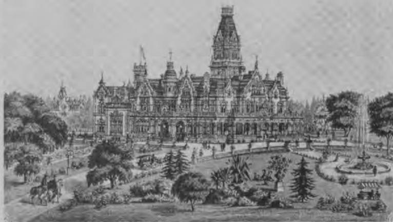
Flood estate, 'Linden Towers' (Britton & Reyes)
