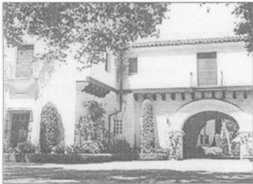
The Jackling House (1925) (website photo).
