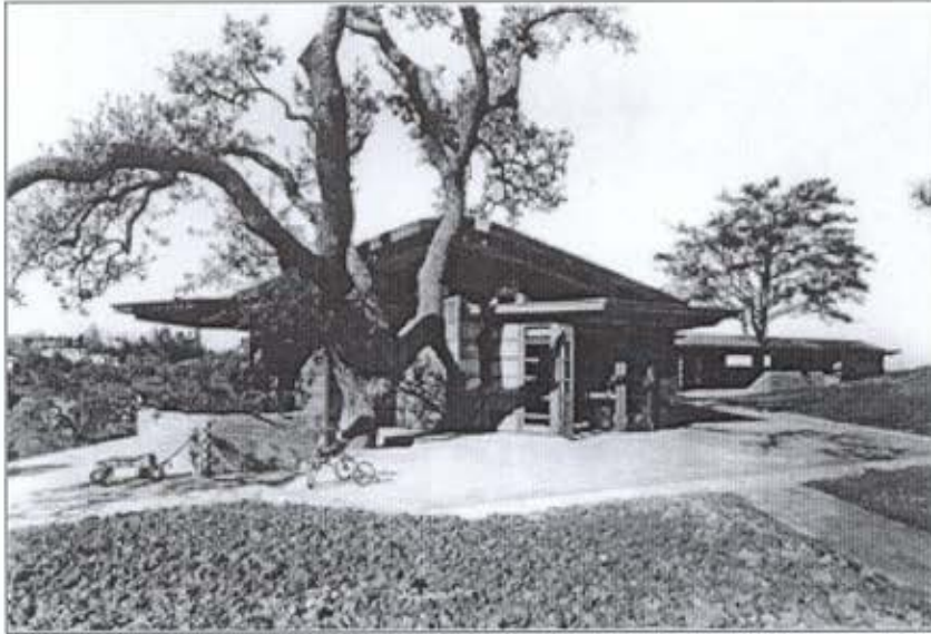
Hanna House as photographed by Esther Born for the Architectural Record, July 1938. Note the Monterey cypress at right rear with carport enclosing it. The valley oak at left is outside daughter Emily-Jean Hanna's bedroom.
