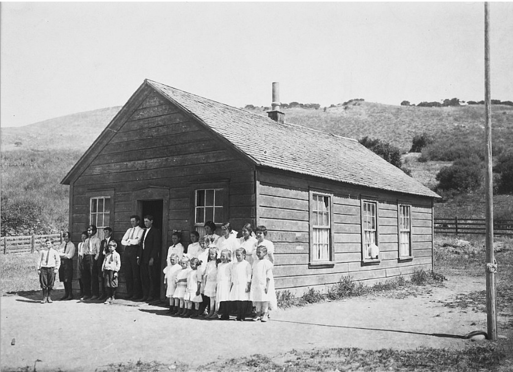
Above: Carmelo School in 1916. The Manor is on the hill beyond the fence. Photo: Monterey County Free Library Local History Collection.
