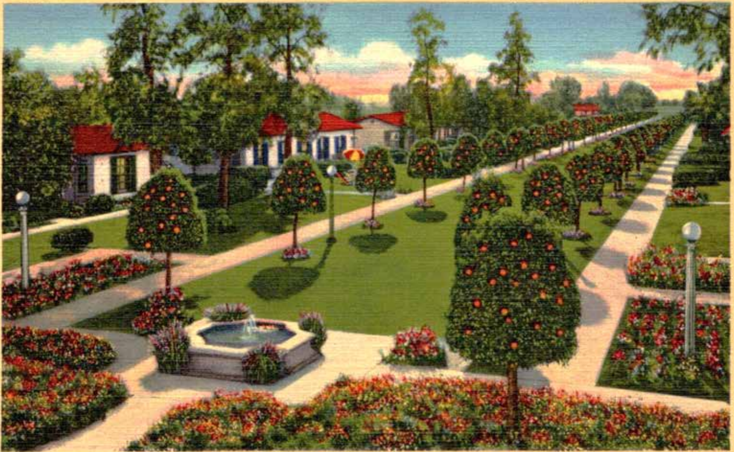
D-15 Orange Vista and Gardens, San Marcos Hotel and Bungalows, Chandler, Arizona
