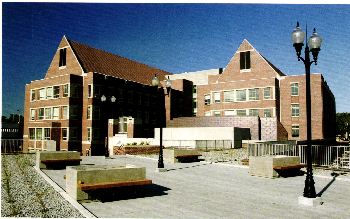
The east façade, above, clearly shows the design concept of two rectangular parallel “bars” linked by the stairway (below) element. Photo shows plaza deck and green roof over the vivarium.
