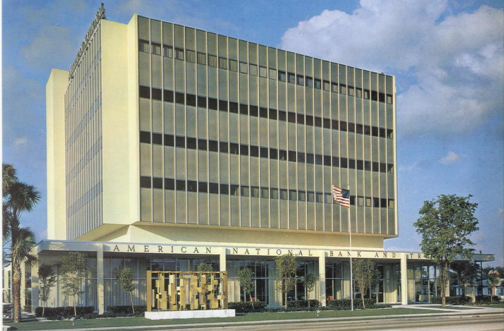
Look of simplicity of Fort Lauderdale bank building a goal achieved with careful planning. Growth plan will accommodate future floors.
