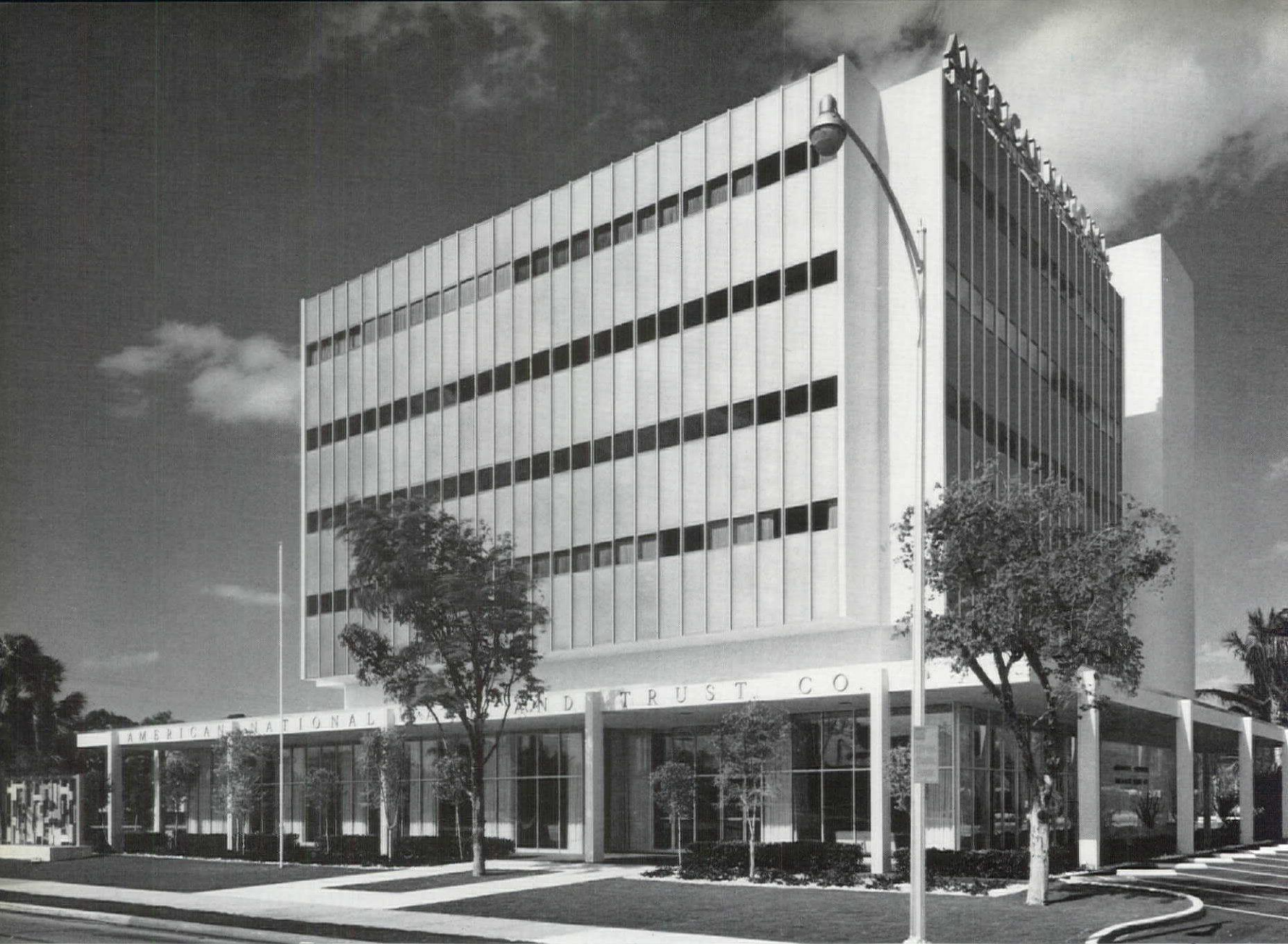
Covered walkway around main banking area of American National's new building keeps lighting bright and pleasant within.
