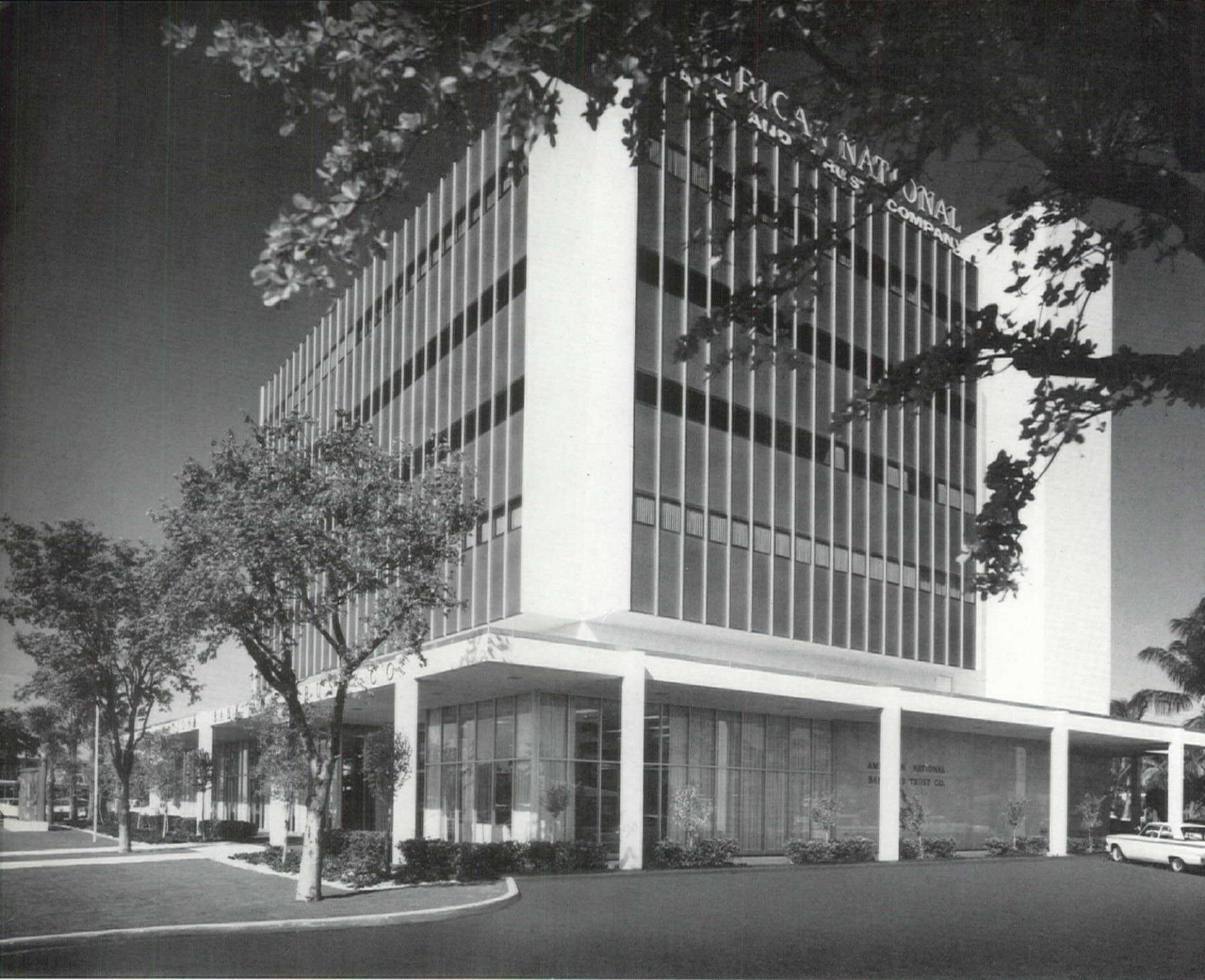
The new American National Bank & Trust Company, Fort Lauderdale, Florida. William T. Vaughn, Architect—Mitchell-Gordon Associates, Consulting Engineers
