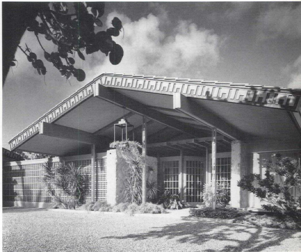
Entry gable facia is enhanced by the application of sculptured wood plaques over oxidized copper.
