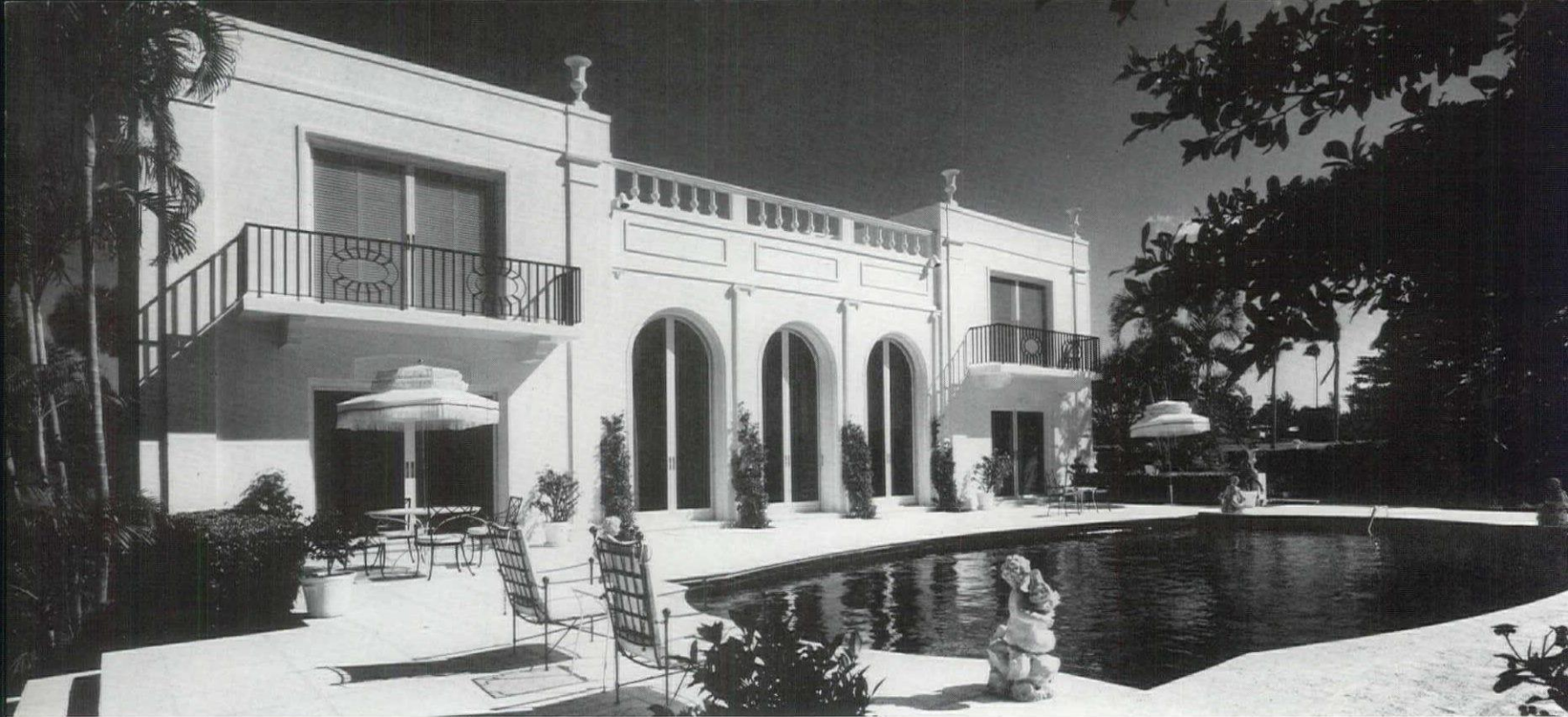
Residence of Mr. and Mrs. Peter I. B. Lavan, North Lake Way, Palm Beach.
