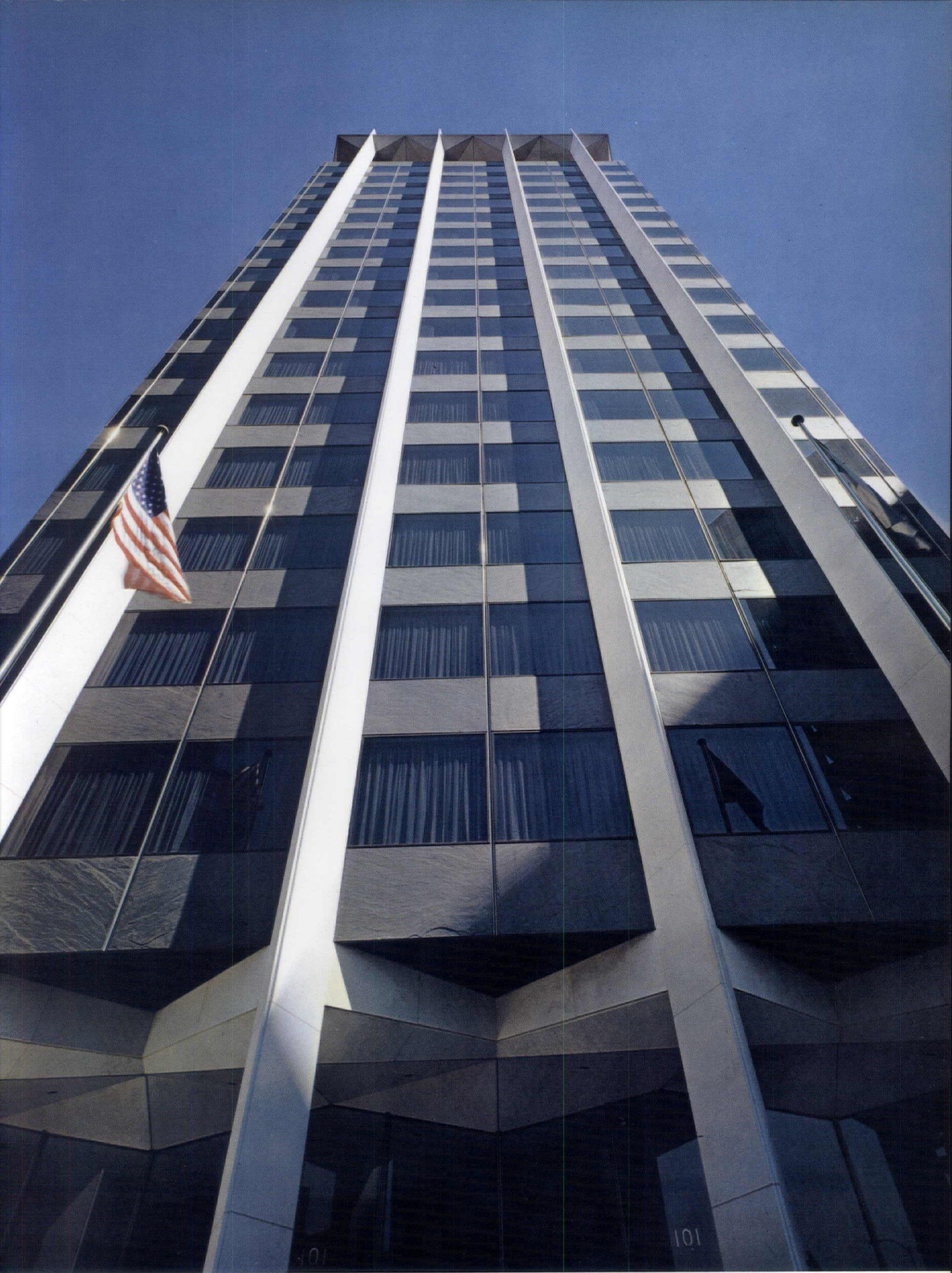
Dramatic effect of white marble dividers against natural slate and blue-tinted glass in upward glance of U. S. Gypsum building.
