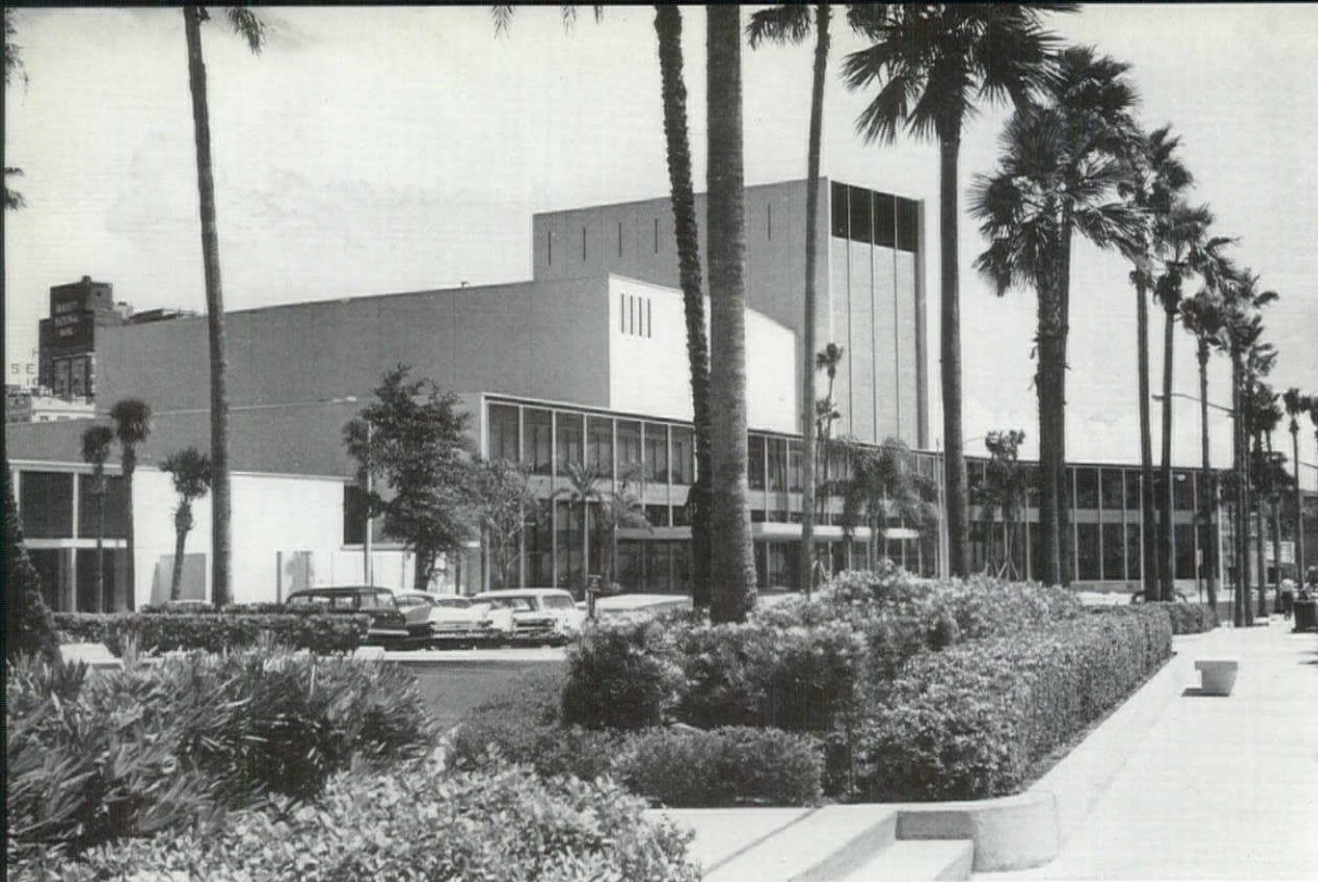
Attractive landscaping enhances the main entrance. Auditorium is an attractive addition to the skyline of Jacksonville.
