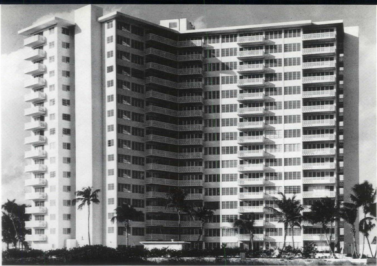
Royal Admiral—Coral Manor Corp., Contractor • Charles F. McKirahan, Architect.
