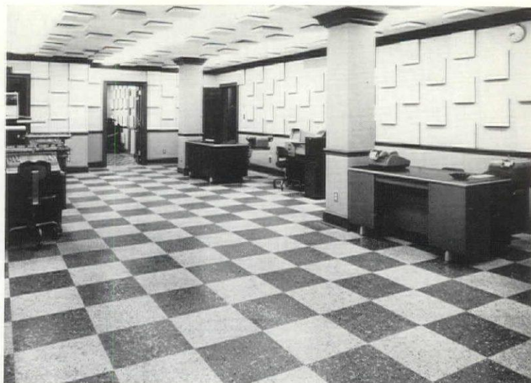
Savings institution boasts rugged \frac{3}{8} " thick Tuflex rubber floor tile . . .
