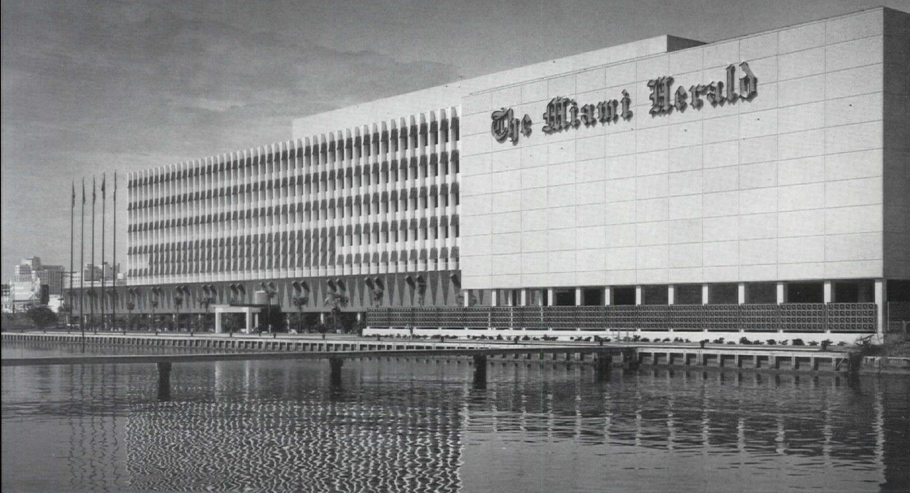
Skillful use of grill screen and three-dimensional concrete panels give massive look to base of building, obscure otherwise floating appearance of open air ground level.
