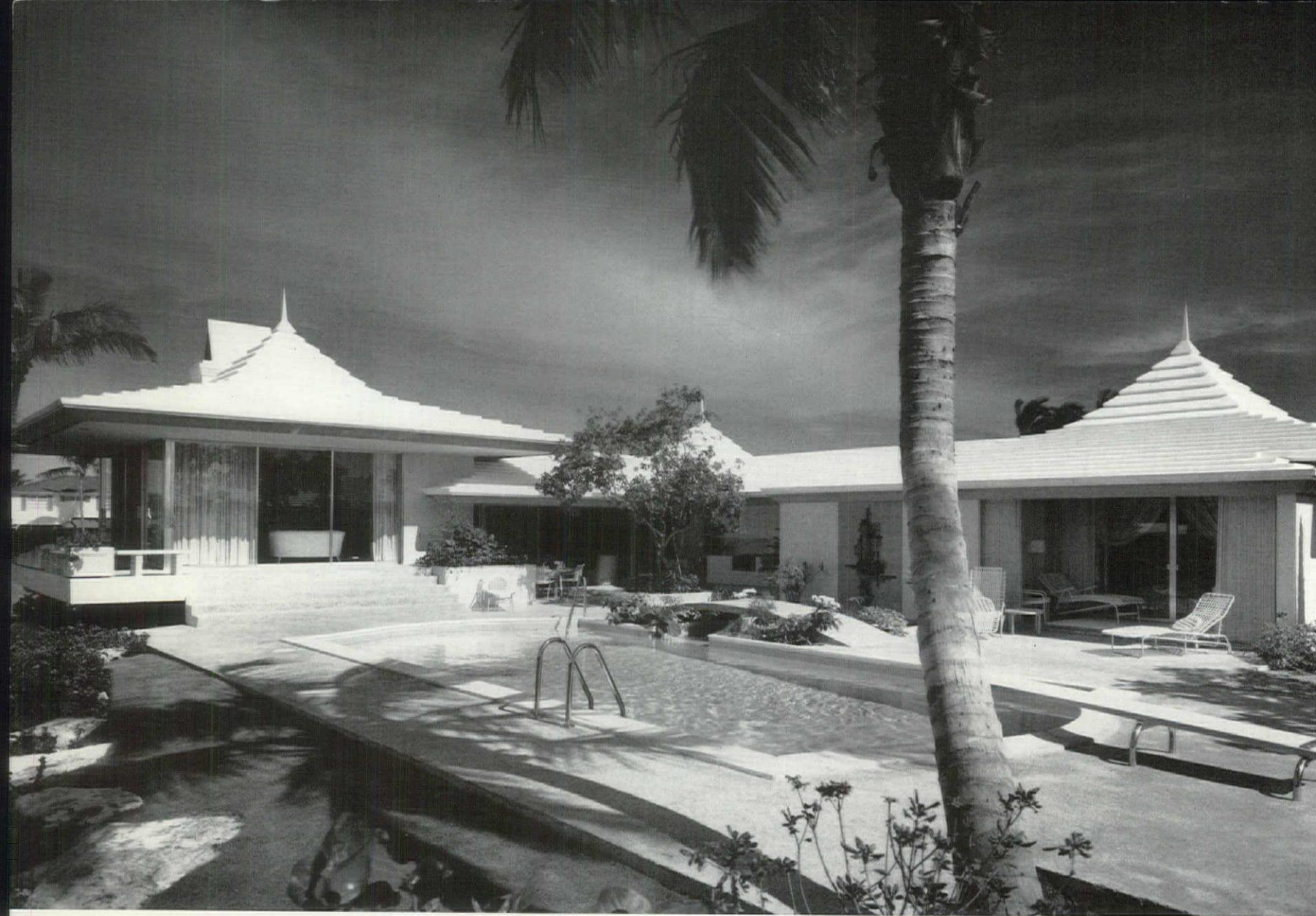
Waterway side of house features pool-patio, central activity center of the home. Barbecue area and ceramic fountain are features.
