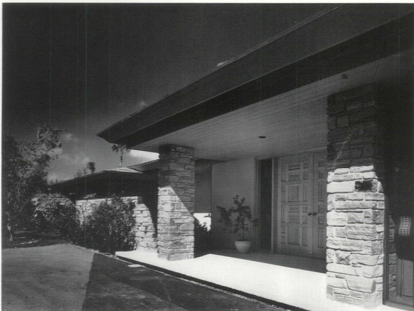
Chesapeake Hue stone piers flank the front entry, featuring a pair of paneled cypress doors.
