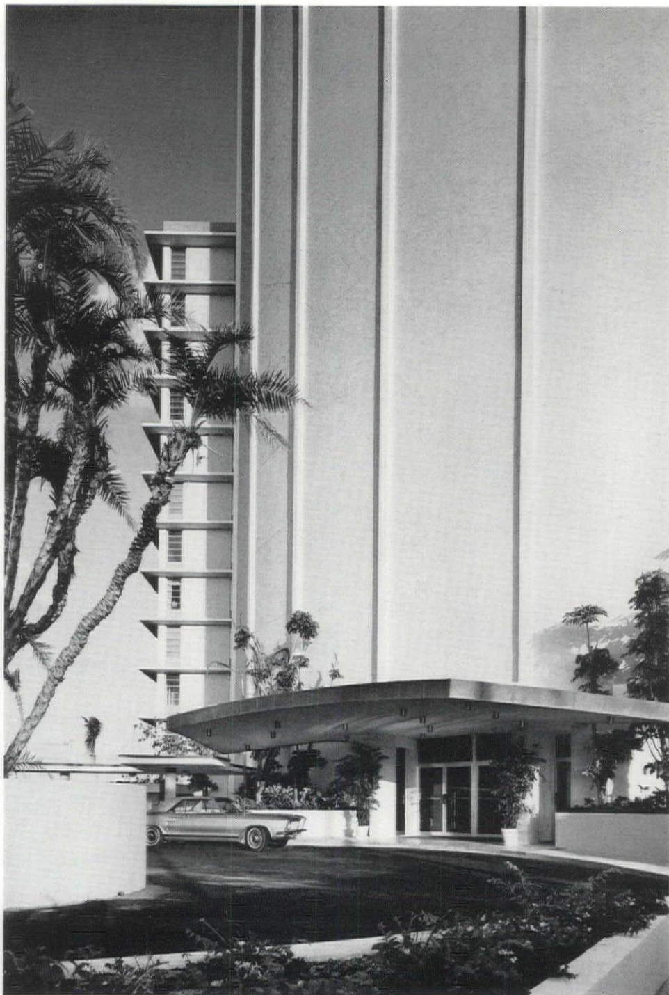
The elevated parking deck features a three-car cantilevered entrance canopy and raised planting areas.
