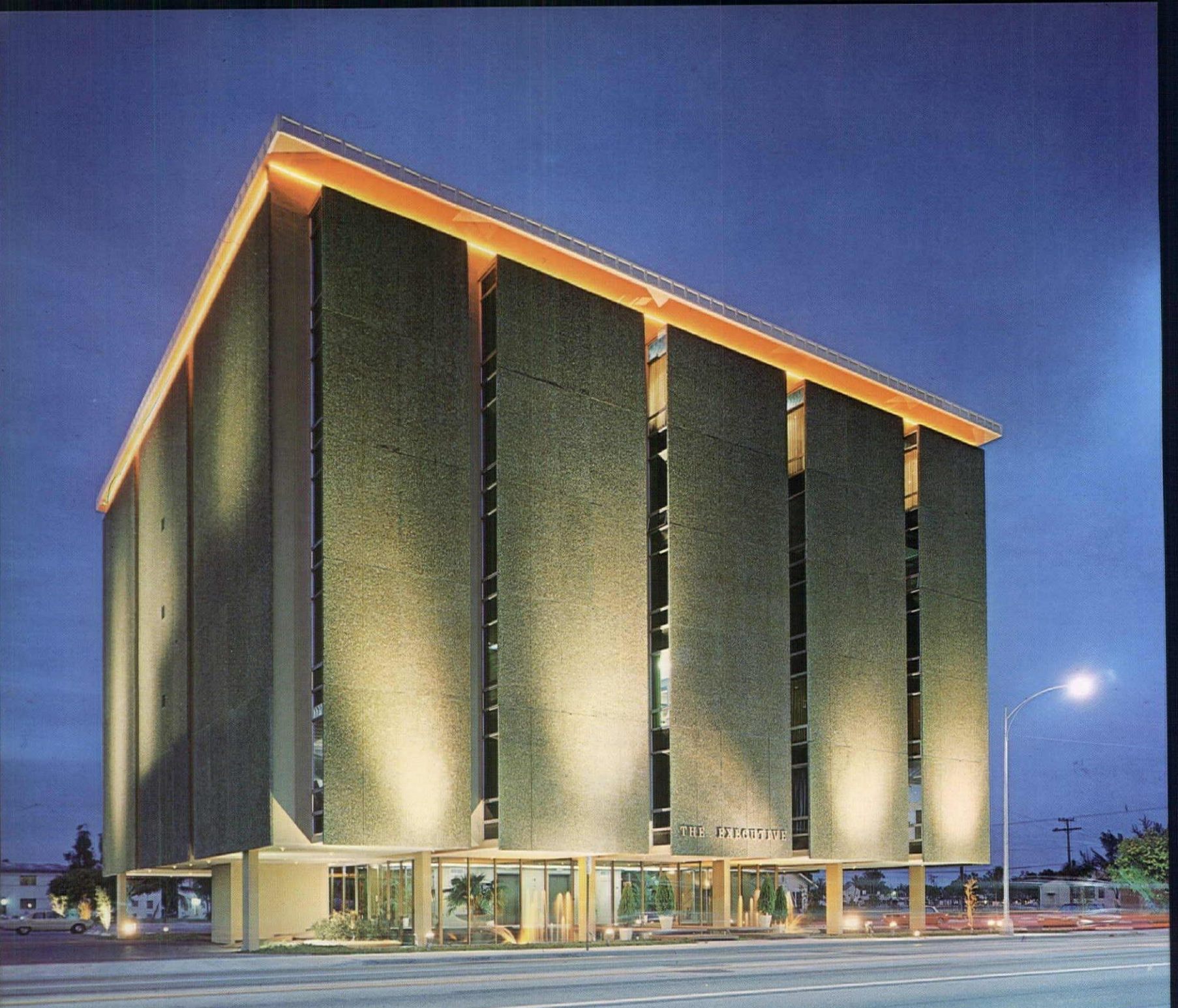
After-dark light play on pre-cast aggregate panels gives illusion of glittering jade. Glass-enclosed entrance lobby allows freedom of movement and attitude.
