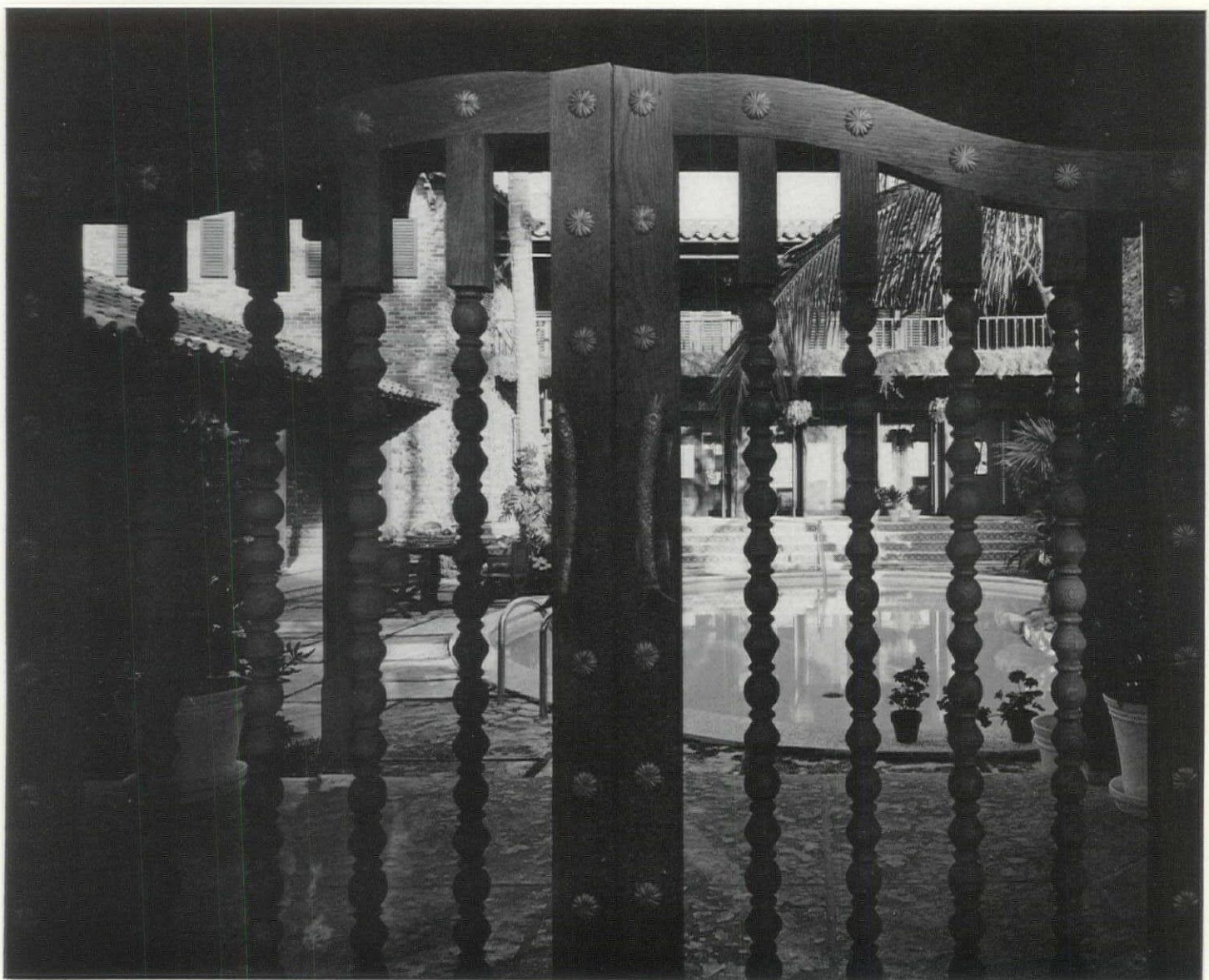
Covered entrance to the courtyard area, showing the use of rough beams, weathered materials and hand-turned spindles.
