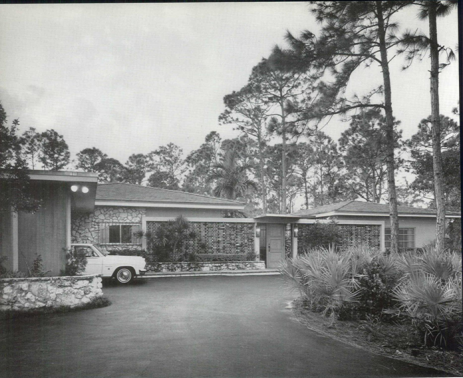
Main entrance garden is enclosed by aged brick grille. Native keystone forms planters.
