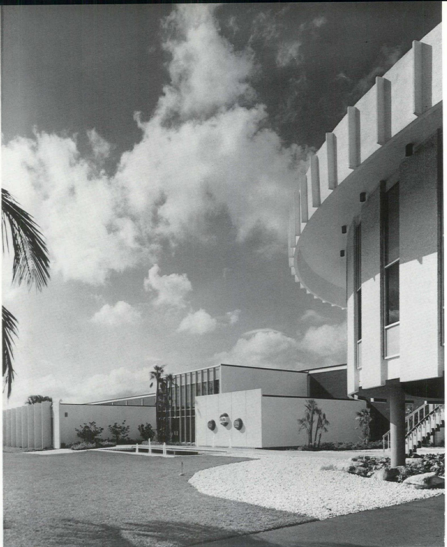
The main entrance remains in keeping with the modern concept of the age. Office areas, below, are sun-controlled by precast concrete panels.
