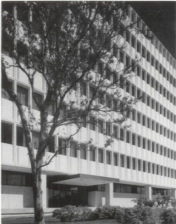
Parking lot is reached from main entrance by protected walkway.
