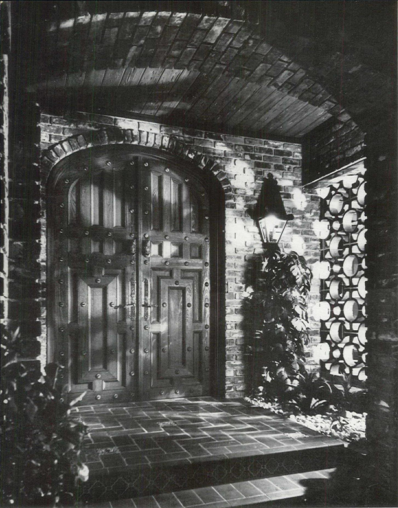
The main house entrance with its magnificent pair of Spanish doors. These doors were found on an estate in southern Spain and sent back to Florida and restored. Some three inches thick, they set the tone of the residence with their feeling of rugged strength, warmth and mellowness. The doors and entry are set off by a planting area and pierced grill wall to filter the sun.
