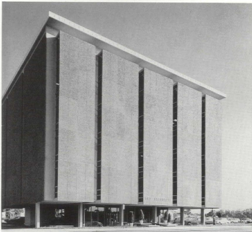
Front facade of building showing main entrance across moat-like mirror pool to main lobby.
