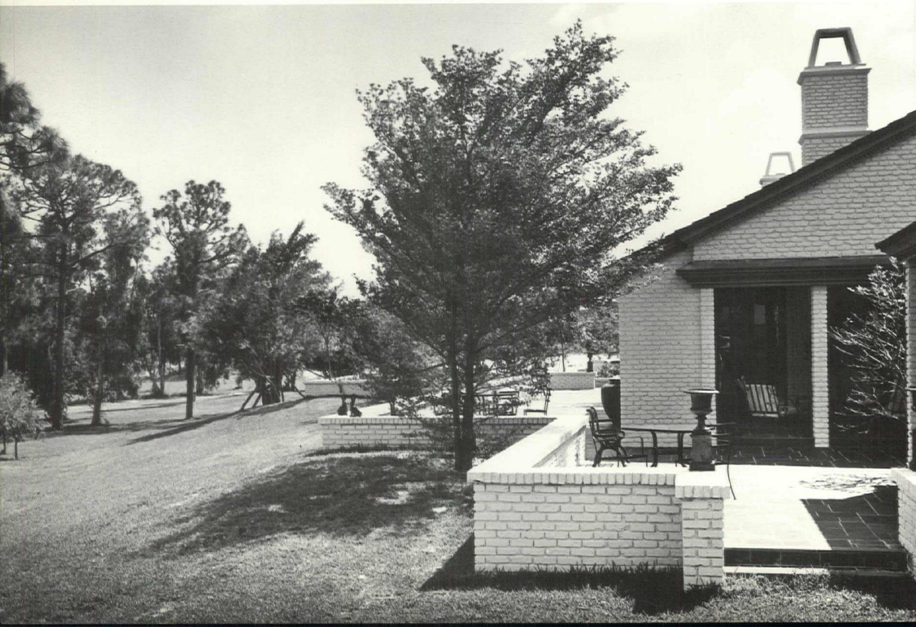
The broken contour of the terrace retaining wall provides private terrace from guest bedroom.
