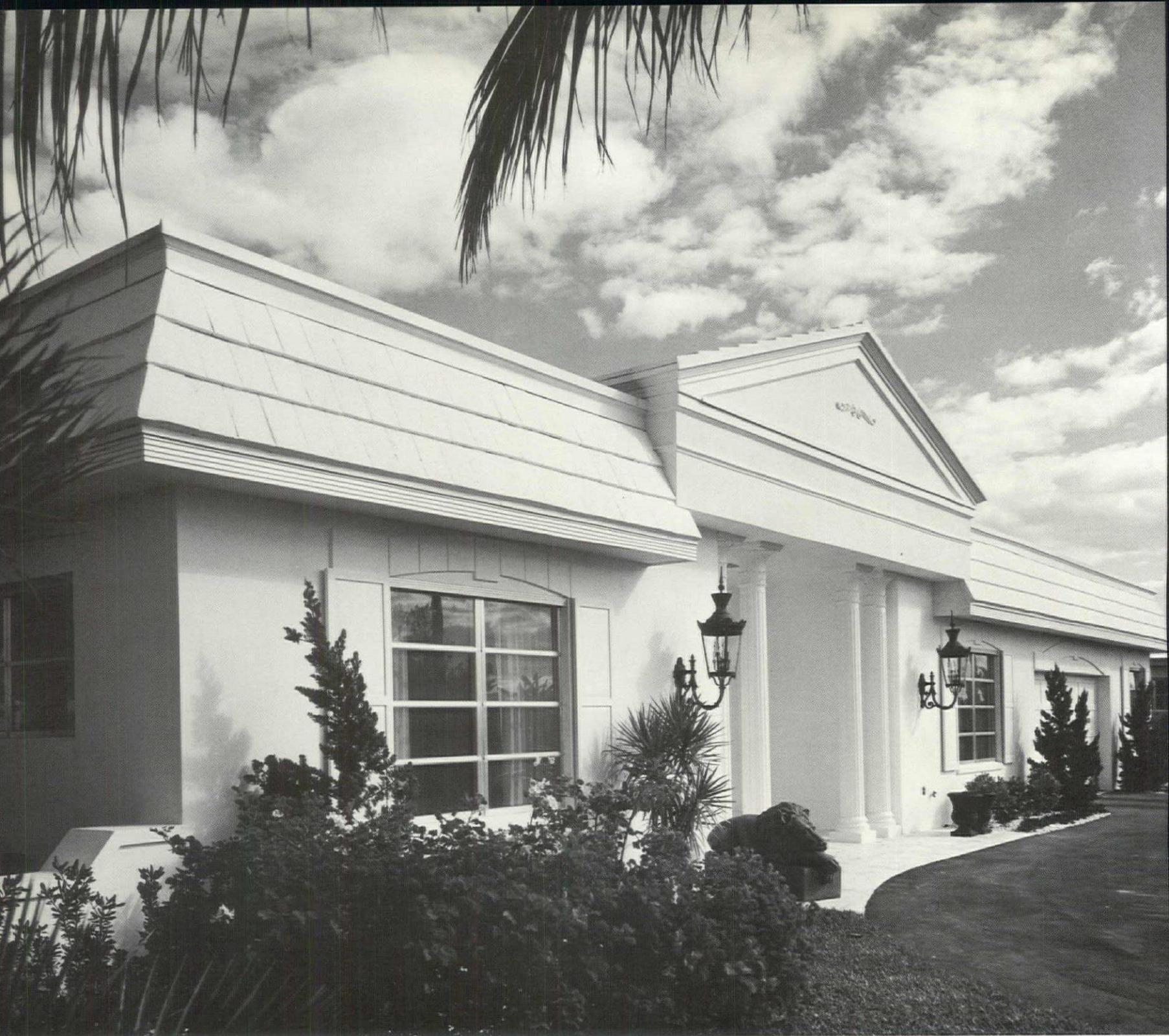
A lion sculpture, two formal urns, and a pair of handsome French lanterns decorate the entrance to the classic lines of the architecture.
