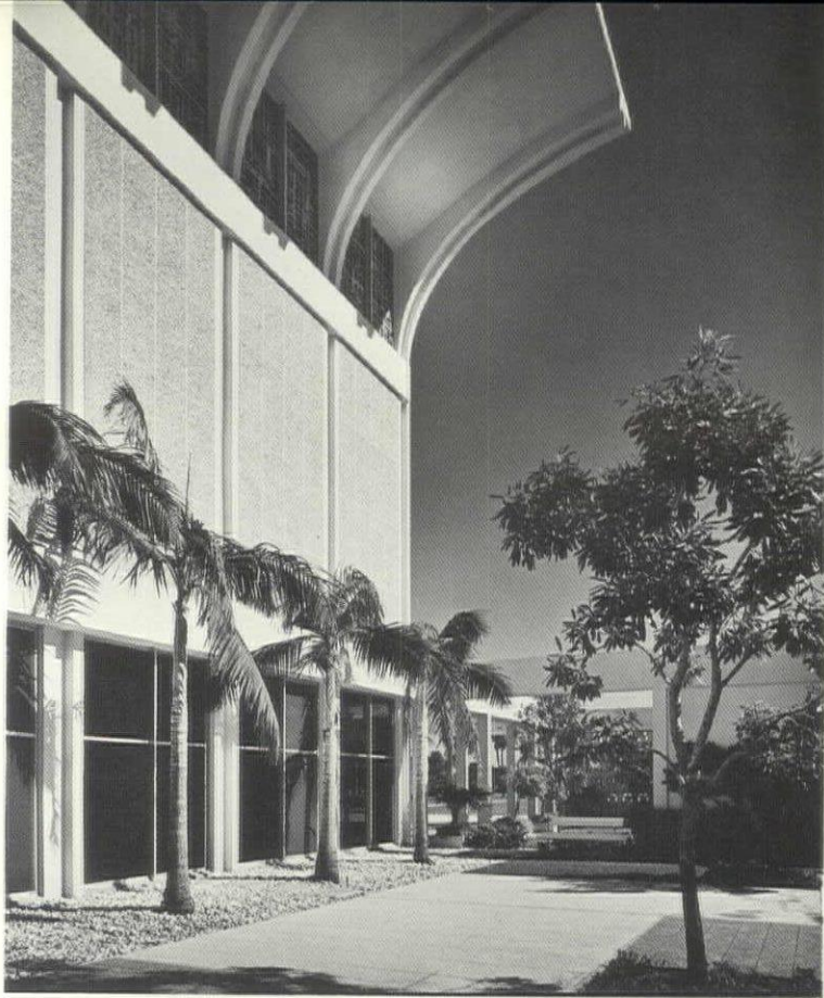
High nave seems to spring to heaven on soaring elements.
