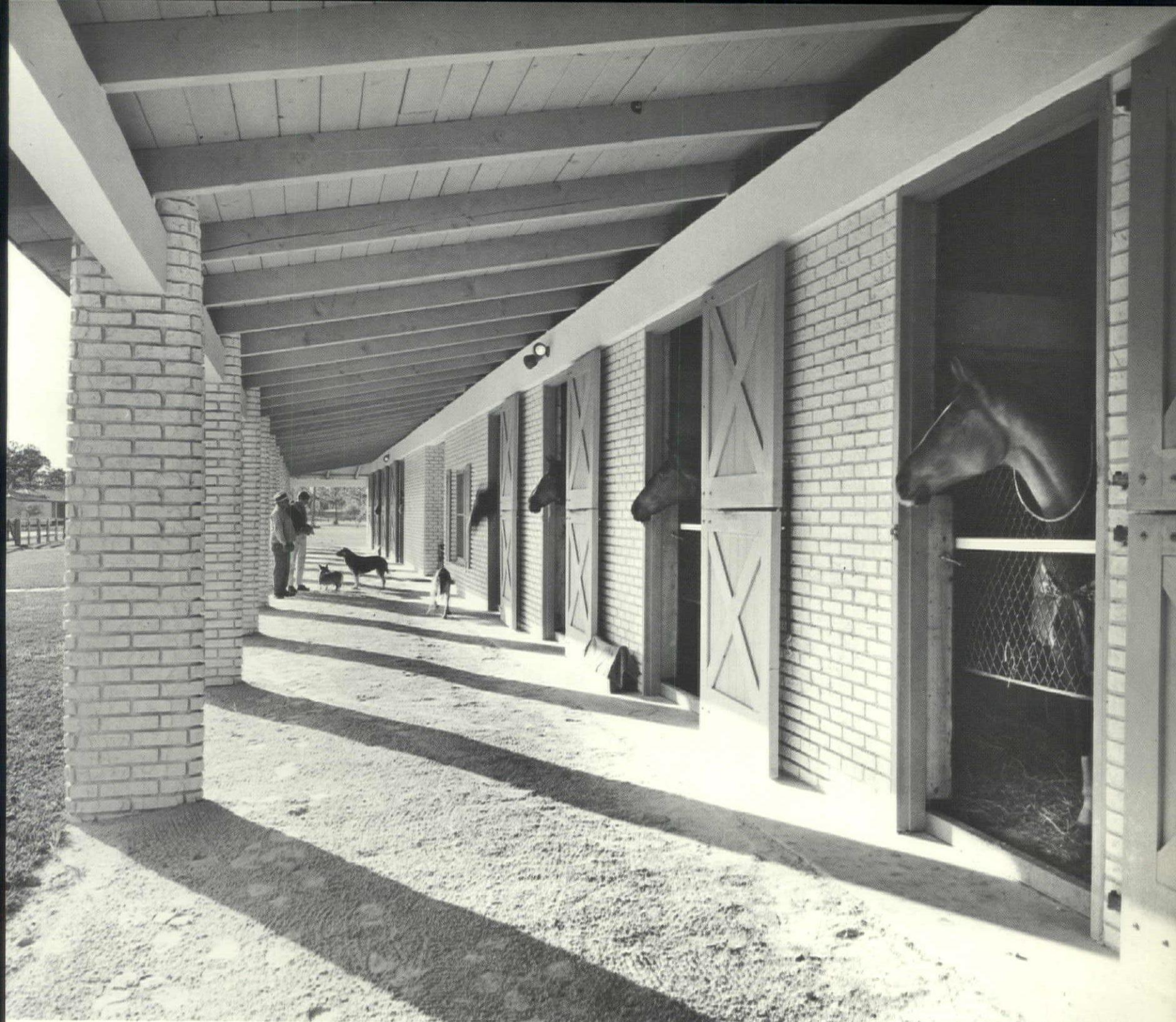
Wide roof overhang of stable shades stalls from late afternoon sun. Across the service drive is manager's residence.
