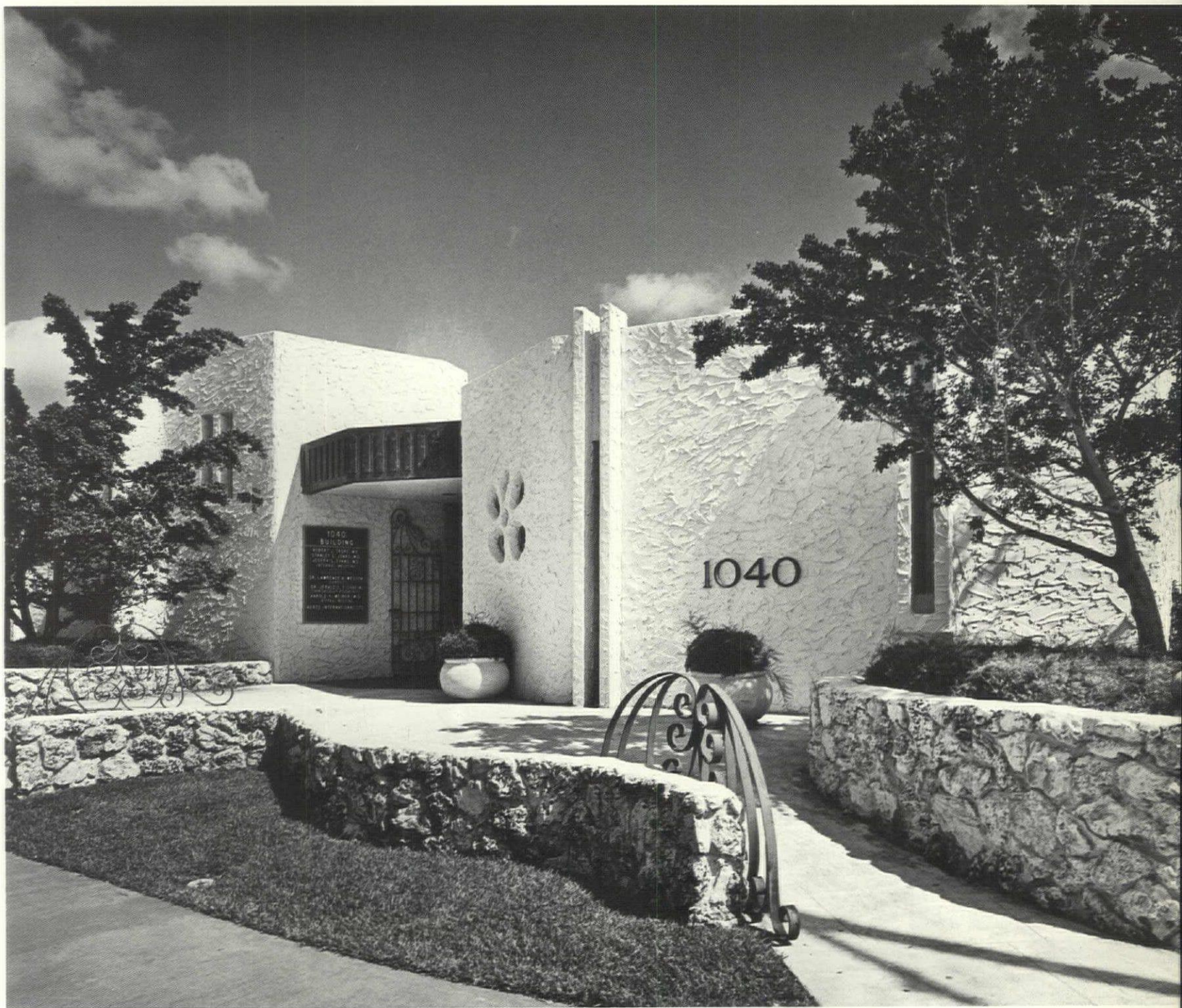
Coral rock retaining walls give a base to the building. Wrought iron railing decorative.
