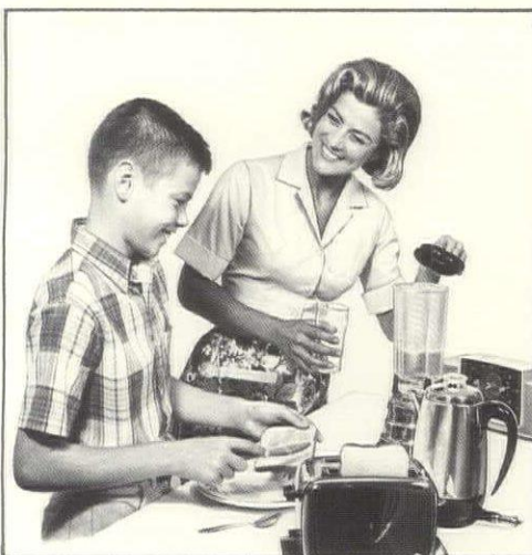
Full Housepower wiring with plenty of handy switches and outlets.
