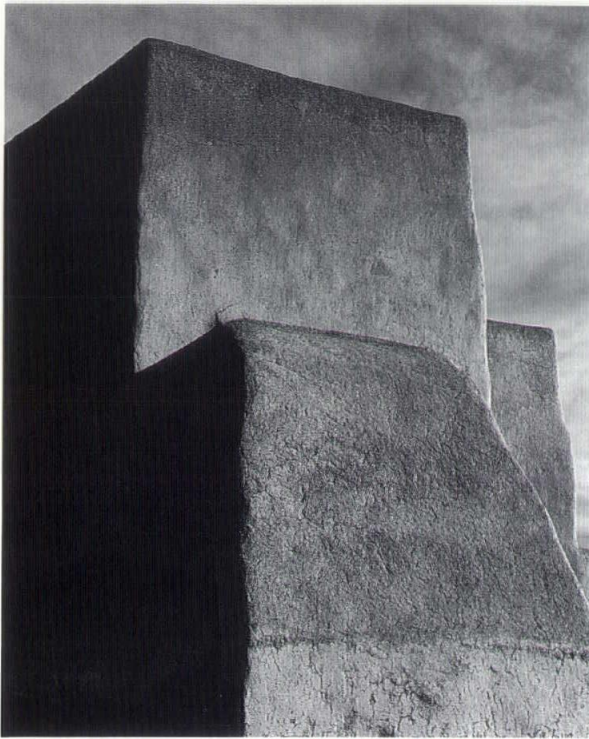
Buttresses at San Francisco de Asisi, Ranchos de Taos, New Mexico. Const. date 1810.
