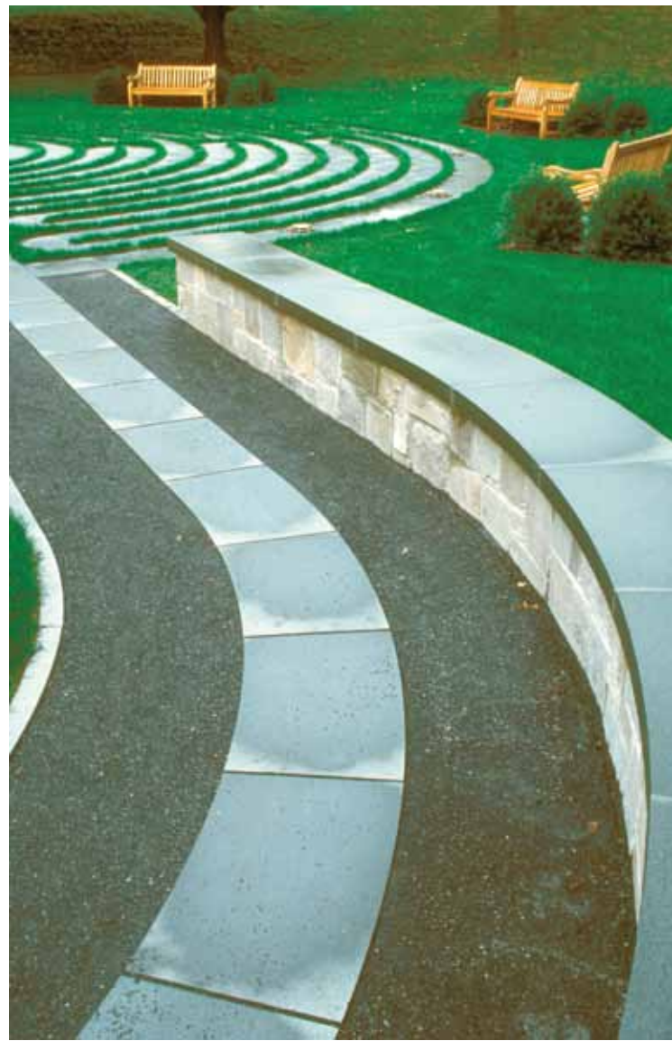
Seatwall, entry path in stone dust field with bluestone edging, and wood benches.
