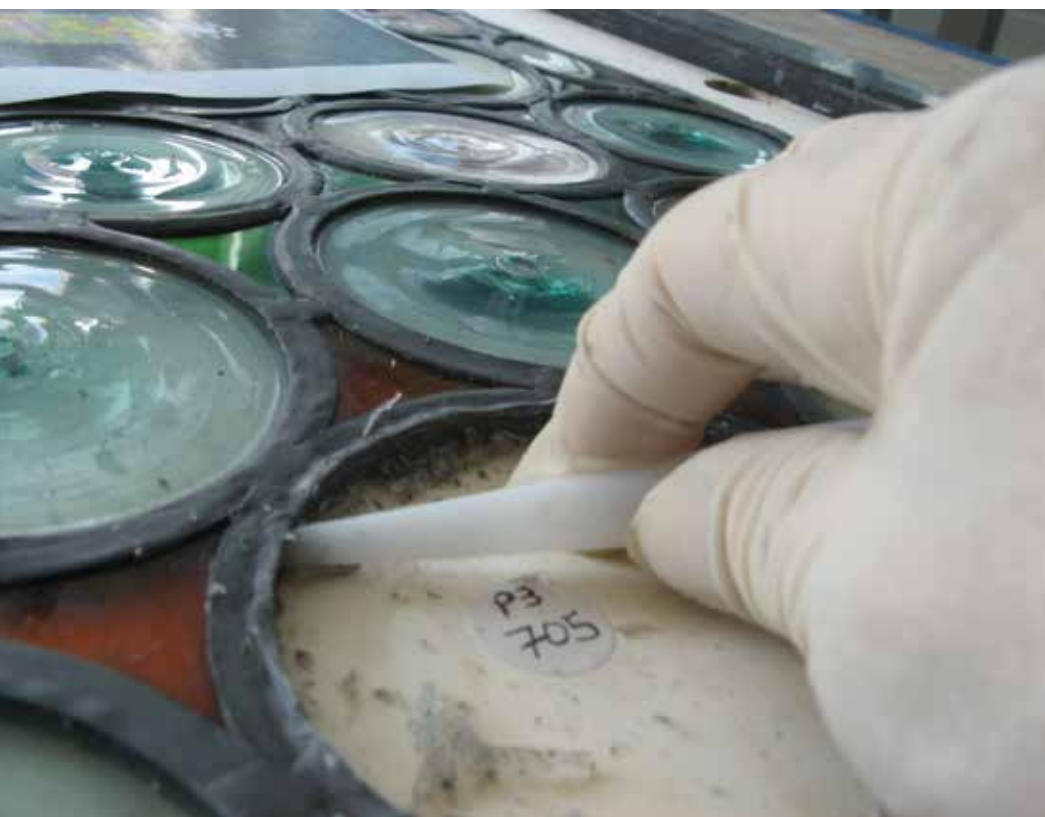
Part of the new restoration involved the removal of inadequate restoration attempts from years earlier.
