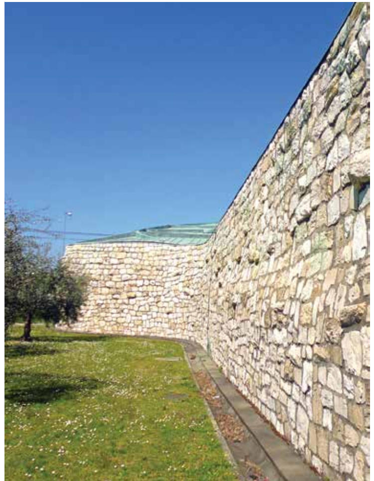
Exterior detail expresses the church's robust construction of rubble stone and copper roofing.
