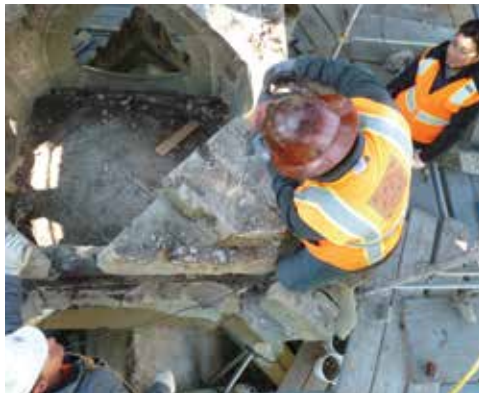
Selective demolition of the upper part of the monument made way for stabilization of remaining masonry.
