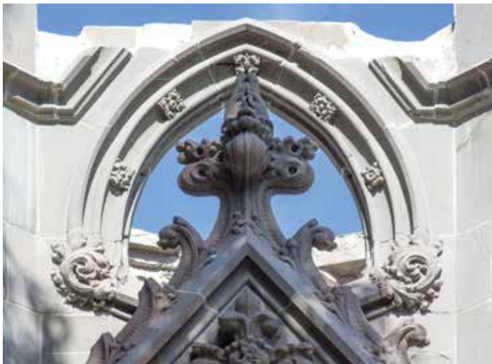
Completed stabilized section of the monument's upper portion; removed masonry has been stored in anticipation of a future complete restoration.
