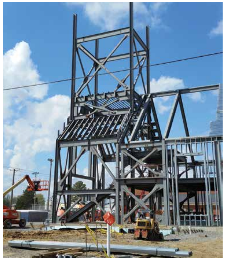
Braced steel framing was used throughout the new church building to increase its wind and earthquake resistance.
