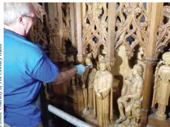
A toothbrush is used to clean the teeth and other details of a figure on the reredos.
