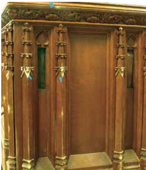
Altar restoration in progress—lighter areas are newly applied bits waiting to be carved and colored.
