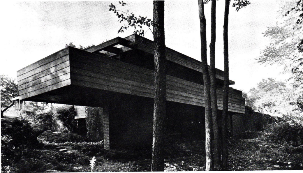
Exterior of Affleck house. The materials are cypress boards and hard burned red brick. Photo courtesy of Balthazar Korab.
