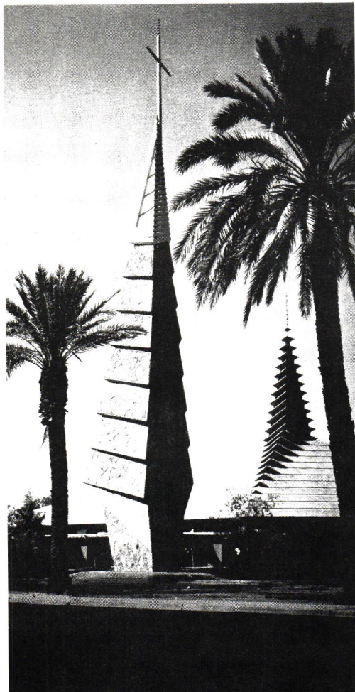
The tower in front completes Wright's design for the site designed in 1957 and completed this year by his successor architectural firm. Photograph courtesy Taliesin.
