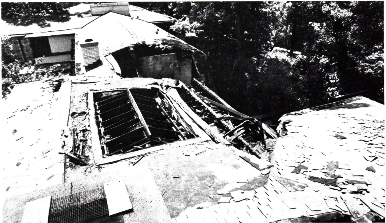
Looking east from the top of the living room chimney showing the extent of the burn. It went east of the fire wall at the center of the photo only about eight feet but went west across the living room and burned through the roof. A small portion of the hole can be seen in the extreme bottom of the photo. Photograph courtesy Thomas A. Heinz.
