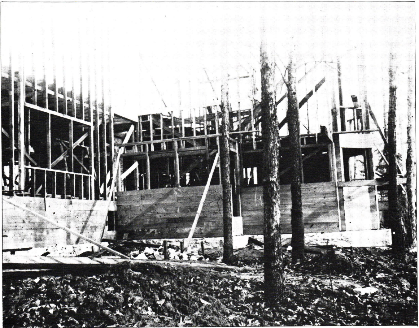
Front south wing of the Willits House during construction, probably during the fall of 1902. The construction is balloon type on a stone foundation that is later covered with a concrete curb. Photo courtesy Peter W. Burnside.
