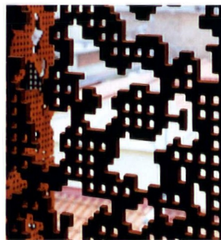
OPPOSITE: The sculptural addition to the Caixa Forum in Madrid reflects the surrounding roofscape. INSET: A detail of the pierced Cor-ten wrapper.
